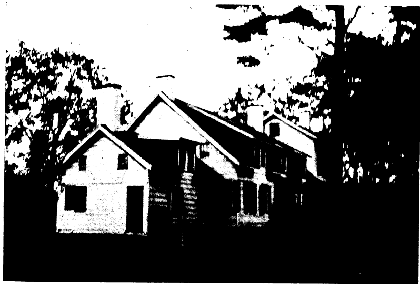
House at South Bound Brook, where Baron Steuben had Quarters and Entertained Washington.
