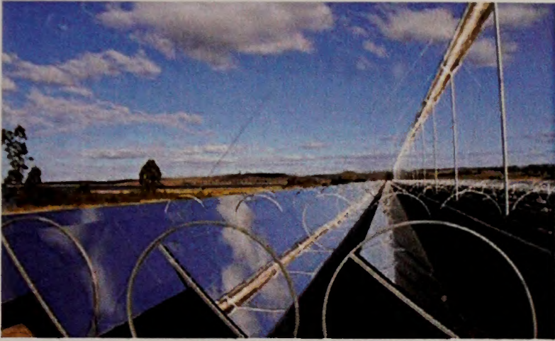
Linear Fresnel technology (Wikipedia.org, Fresnel_reflectors_ausra.jpg)
