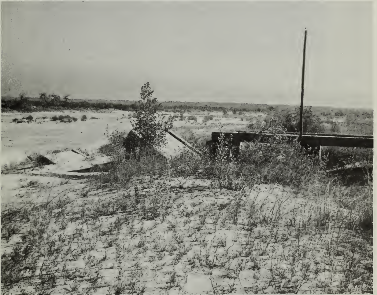
A large flood destroyed this county road bridge near Canadian and left a deep layer of sand on large areas of the flood plain.
