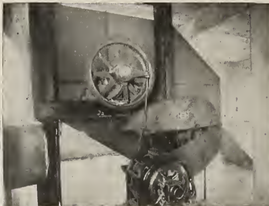
ABOVE: MORSE SILENT CHAIN DRIVE DIRECT TO ELEVATOR HEAD IN FT. WORTH ELEVATORS CO. PLANT, FT. WORTH, TEXAS. LEFT: MORSE SILENT CHAIN DRIVE TO CONVEYOR IN B. & O. ELEVATOR, BALTIMORE, MD. RIGHT: MORSE SILENT CHAIN DRIVE FROM MOTOR TO JACKSHAFT IN SUNSET ELEVATOR, GALVESTON, TEXAS.
