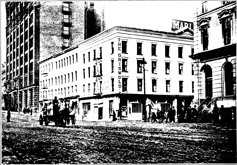
SITE OF UNION TRUST BUILDING IN EARLY '90s The Hammond Building at the left
