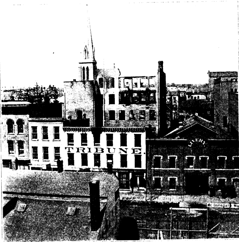
RUINS OF THE DETROIT TRIBUNE BUILDING, APRIL, 1873
