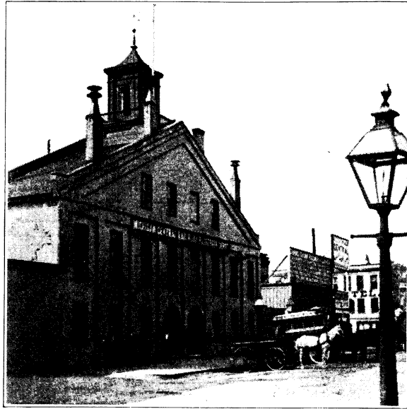
MICHIGAN CENTRAL DEPOT, 1853-83
