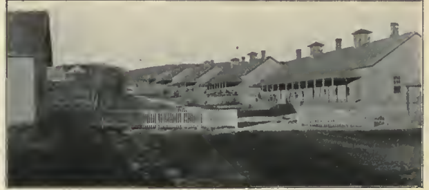
Barrack buildings, and frame cottage on the rise to the north.
