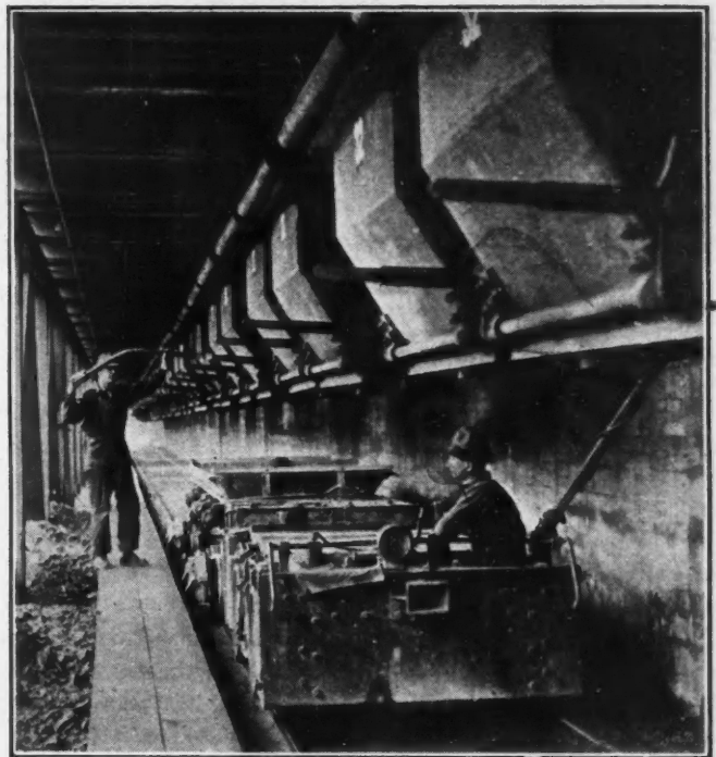
FIG. 16. CHARGING FEED CAR
