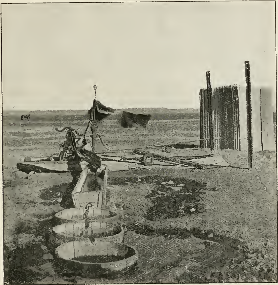
Well with bath and washhouse on one side. These are covered with old galvanized iron, old rail, &c. Tubs where horses and cattle stand and drink. The drainage runs back into the well.
