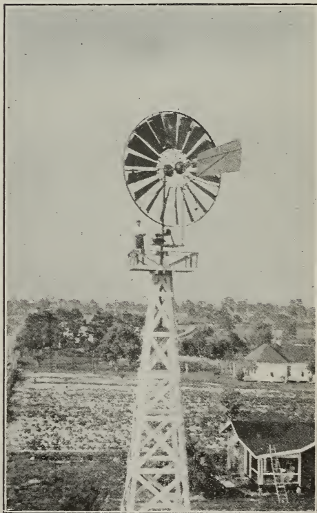
The electric windmill with the builder of the tower (Mr. Leon Wheeler) on the platform, 45 feet up. The highest point of the wheel is 60 feet from the ground.
