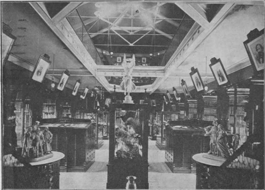
LOWER LIBRARY HALL, IOWA MASONIC LIBRARY, CEDAR RAPIDS
