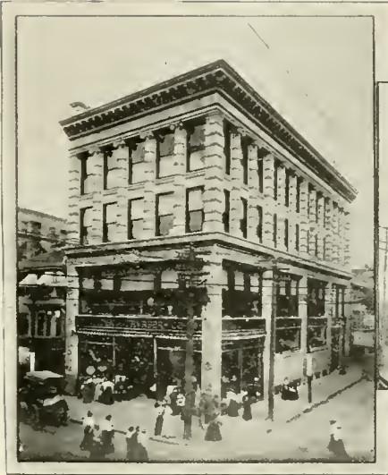
The Tilden & Thurber Co. Building.
