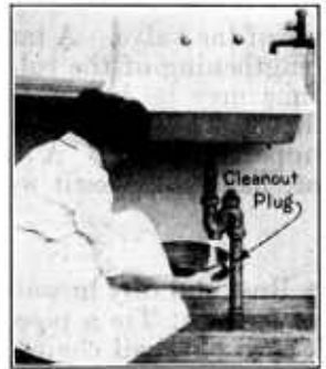
FIG. 9.—Cleaning out a sink trap
