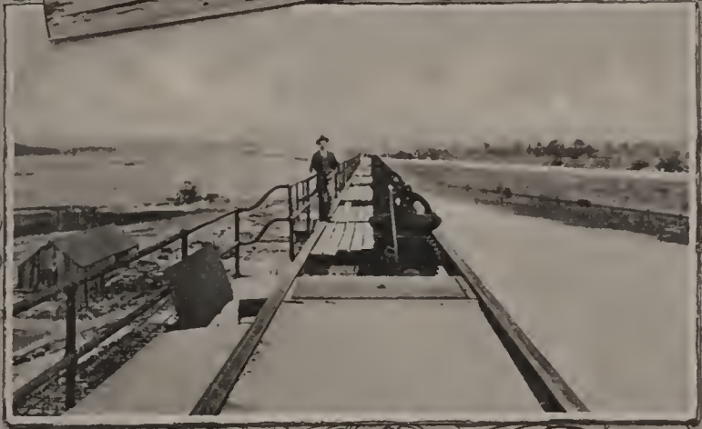
CONTROLLING GEAR OF THE STONEY GATES.
