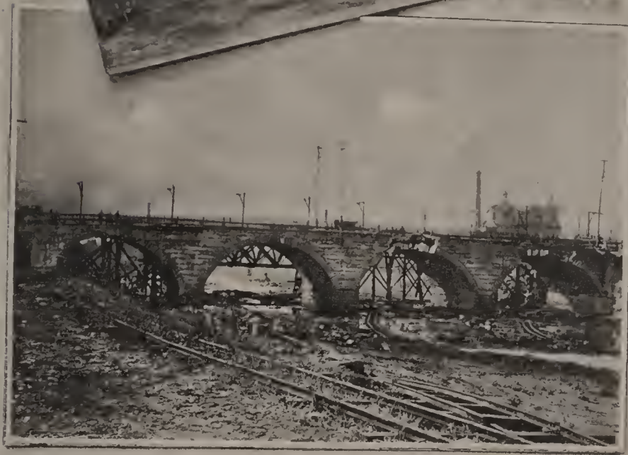
BLOWING UP OF THE JEFFERSON ST. BRIDGE.
