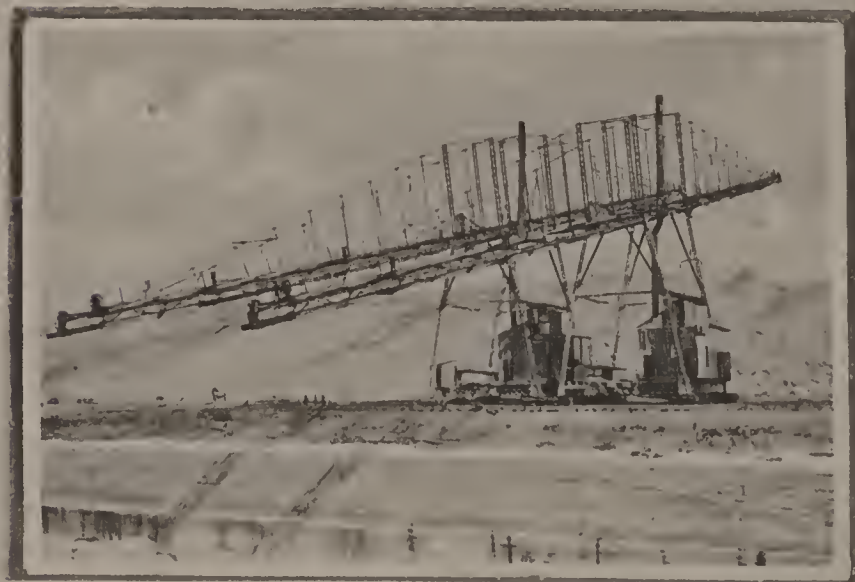
CANTILEVER CONVEYOR 640 FEET LONG.
