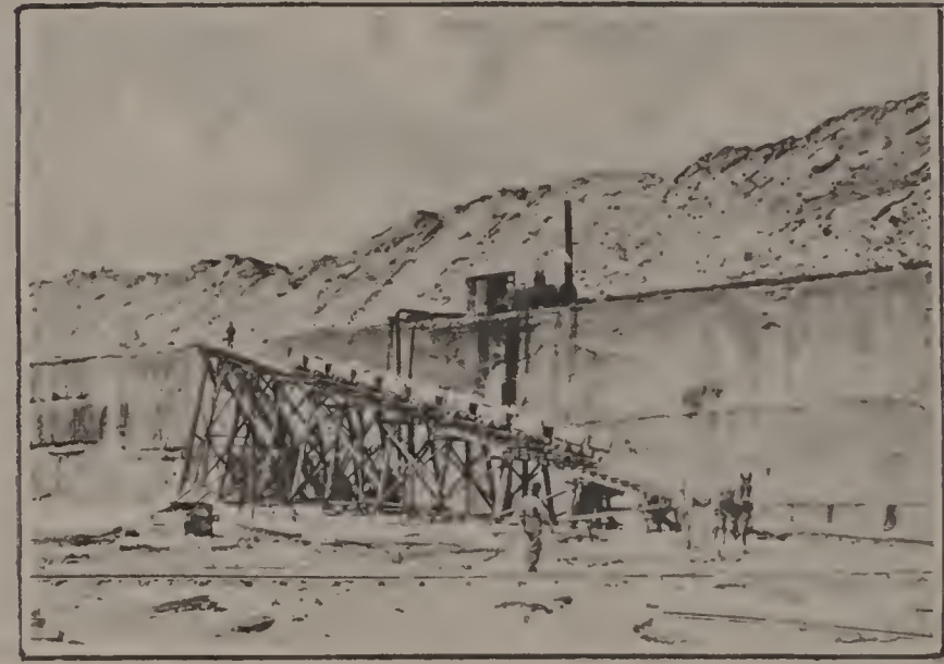
SEC. 9. CABLE TRAMWAY FOR HOISTING CARS.
