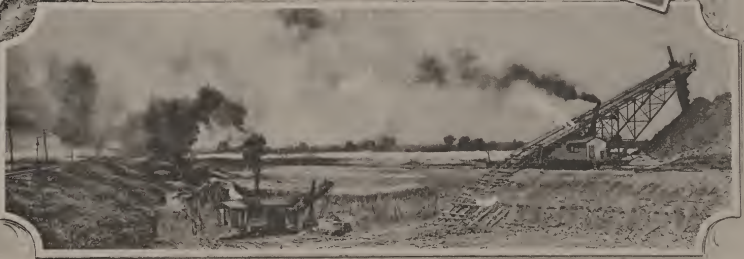
SEC. 5. LIDGERWOOD STEAM DREDGE AND HOIST AT WORK.
