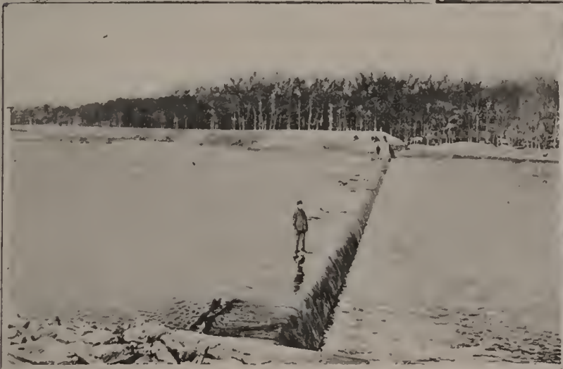
SPILL-WAY DAM AT THE HEAD OF THE NEW DES PLAINES RIVER CHANNEL
