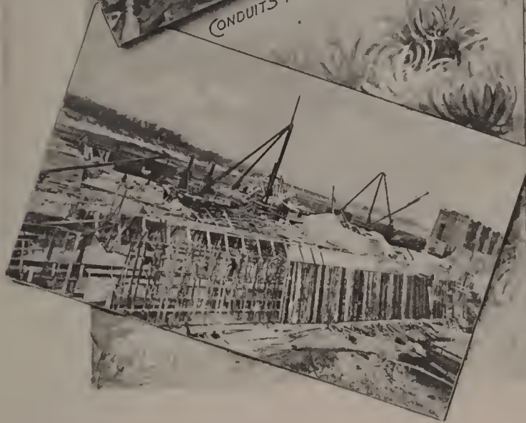
VIEW OF STEEL FRAME WORK FOR DAM.
