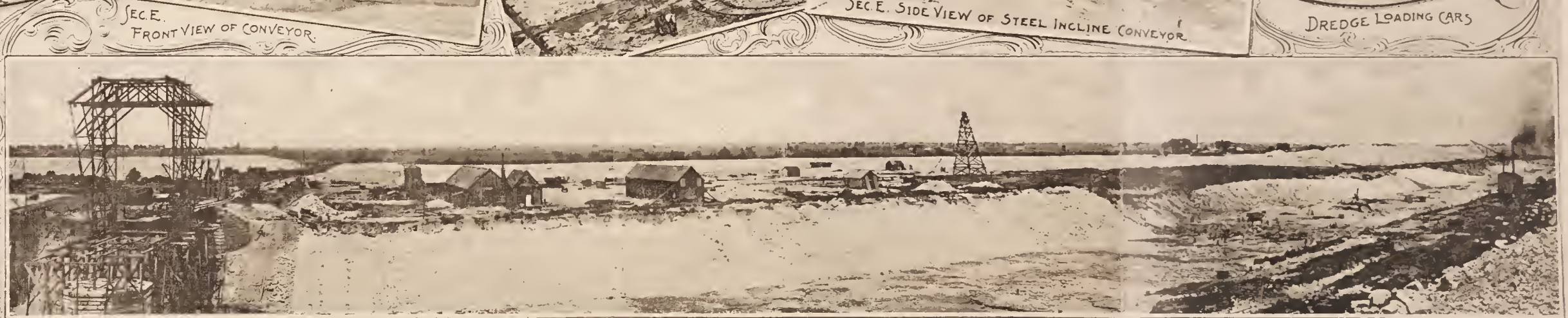
GENERAL VIEW OF SEC. E, SHOWING ABUTMENTS FOR SWING BRIDGE.
