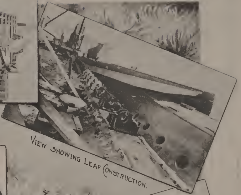
BEAR TRAP DAM NEARING COMPLETION.
