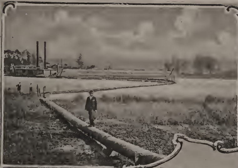
SEC. A & B. HYDRAULIC DREDGE AND PIPE LINE.
