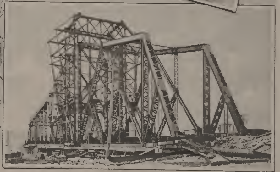
ROLLER TRAMS FOR SPRING BRIDGE.
