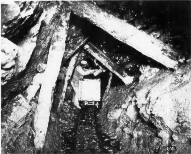
DRIFT, ADIT LEVEL AND CHUTE, JOSEPHINE MINE, COLO.
