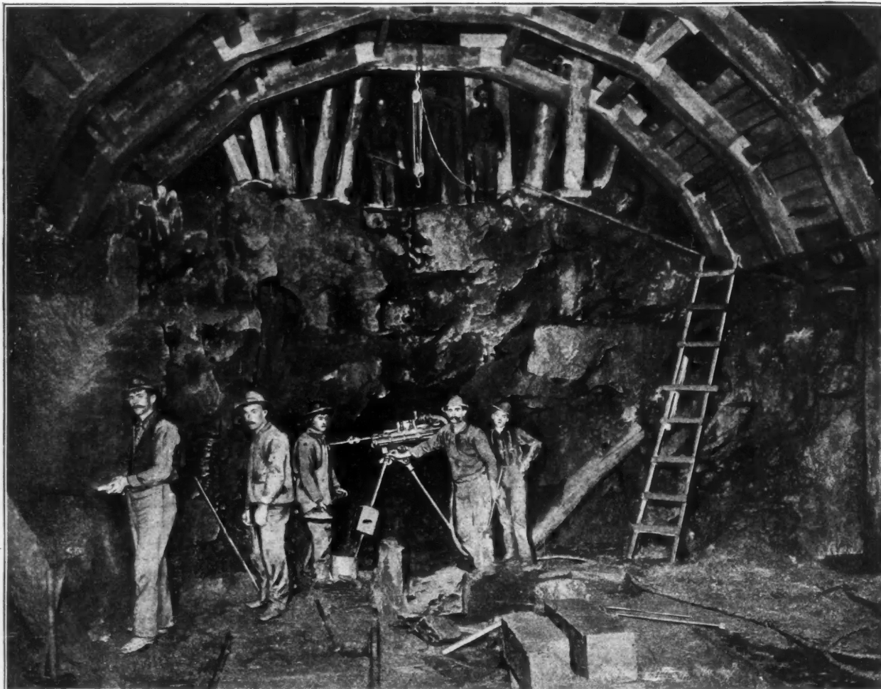
ARCHED TUNNEL IN NEW YORK SUBWAY.
