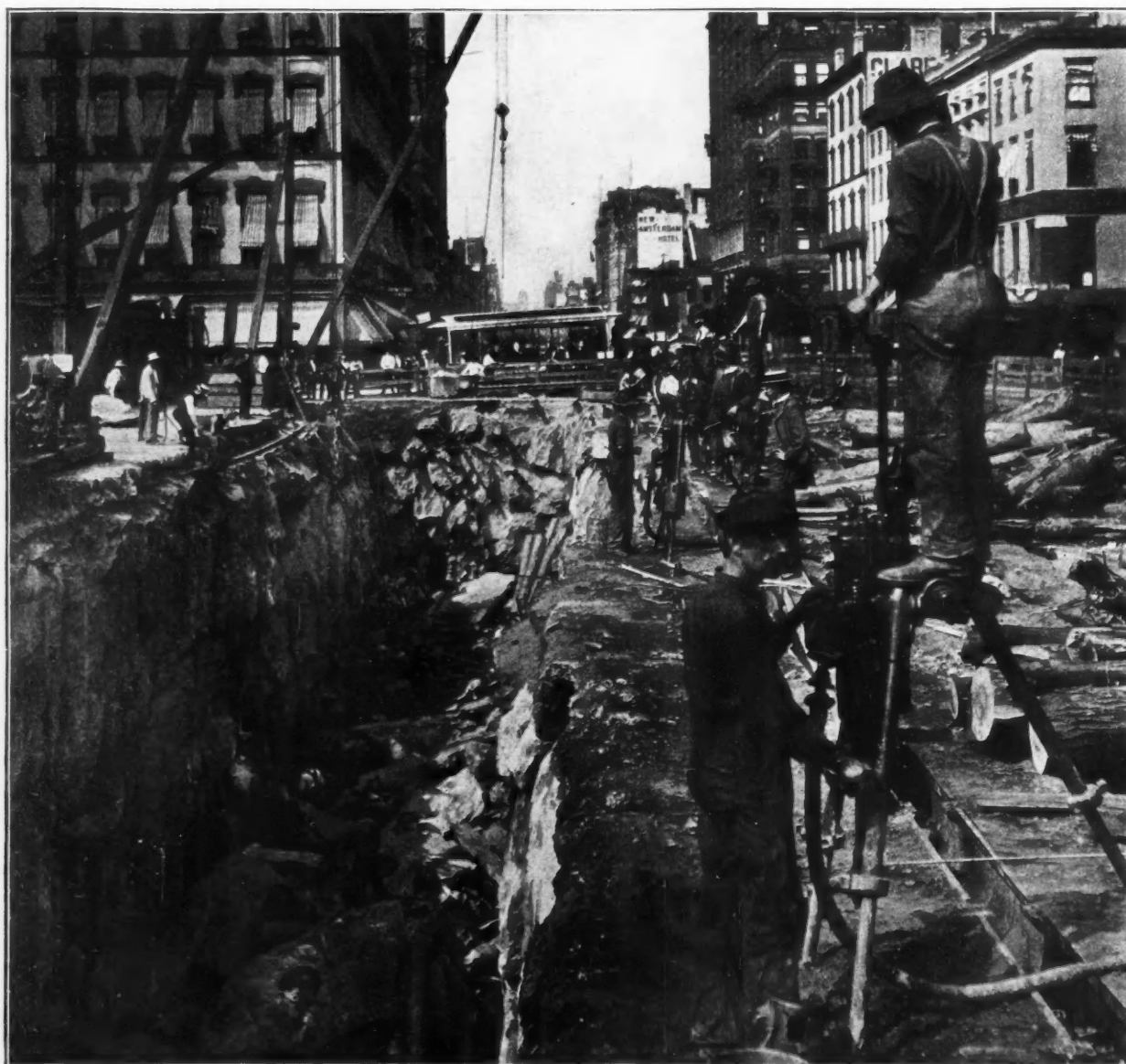
OPEN CUT WORK ON NEW YORK SUBWAY.
