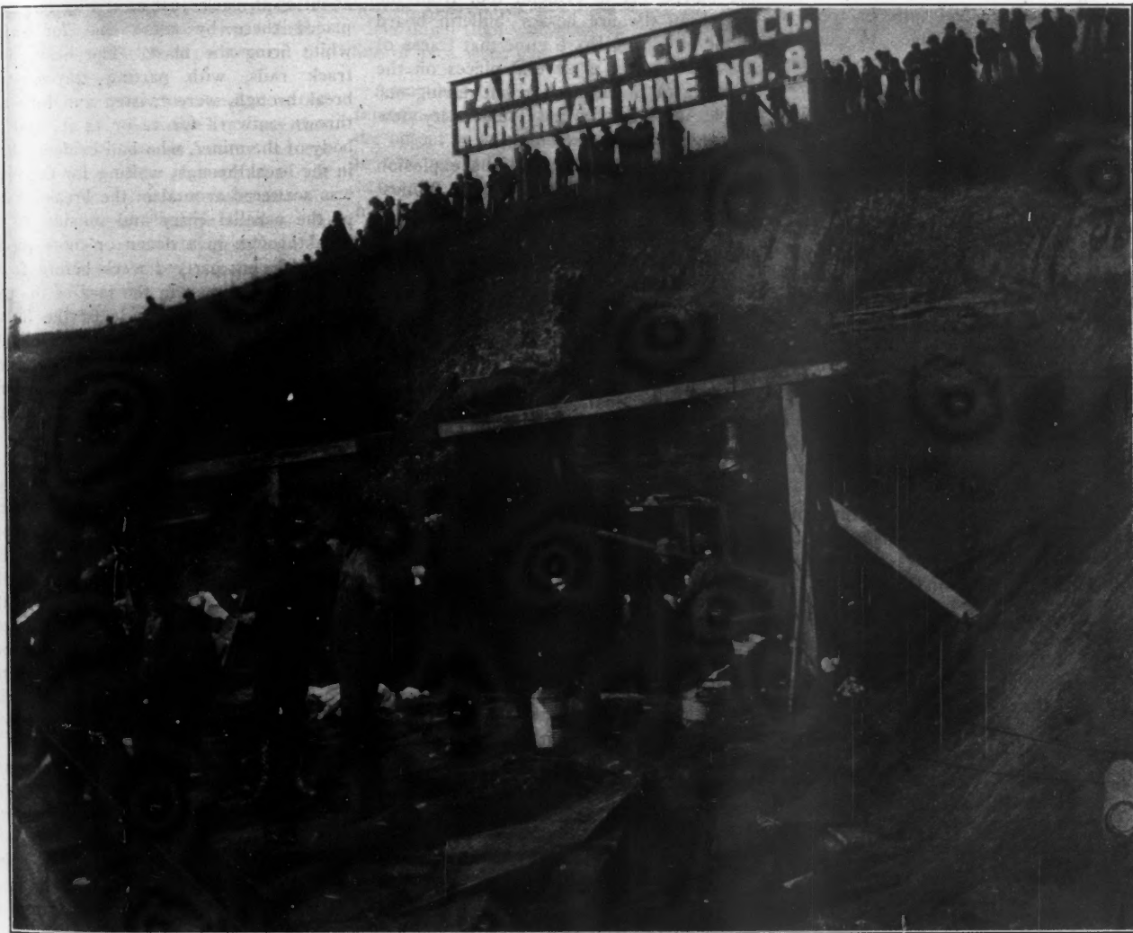
STOPPING UP THE ENTRANCE TO NO. 8, IN ORDER TO RESTORE VENTILATION
