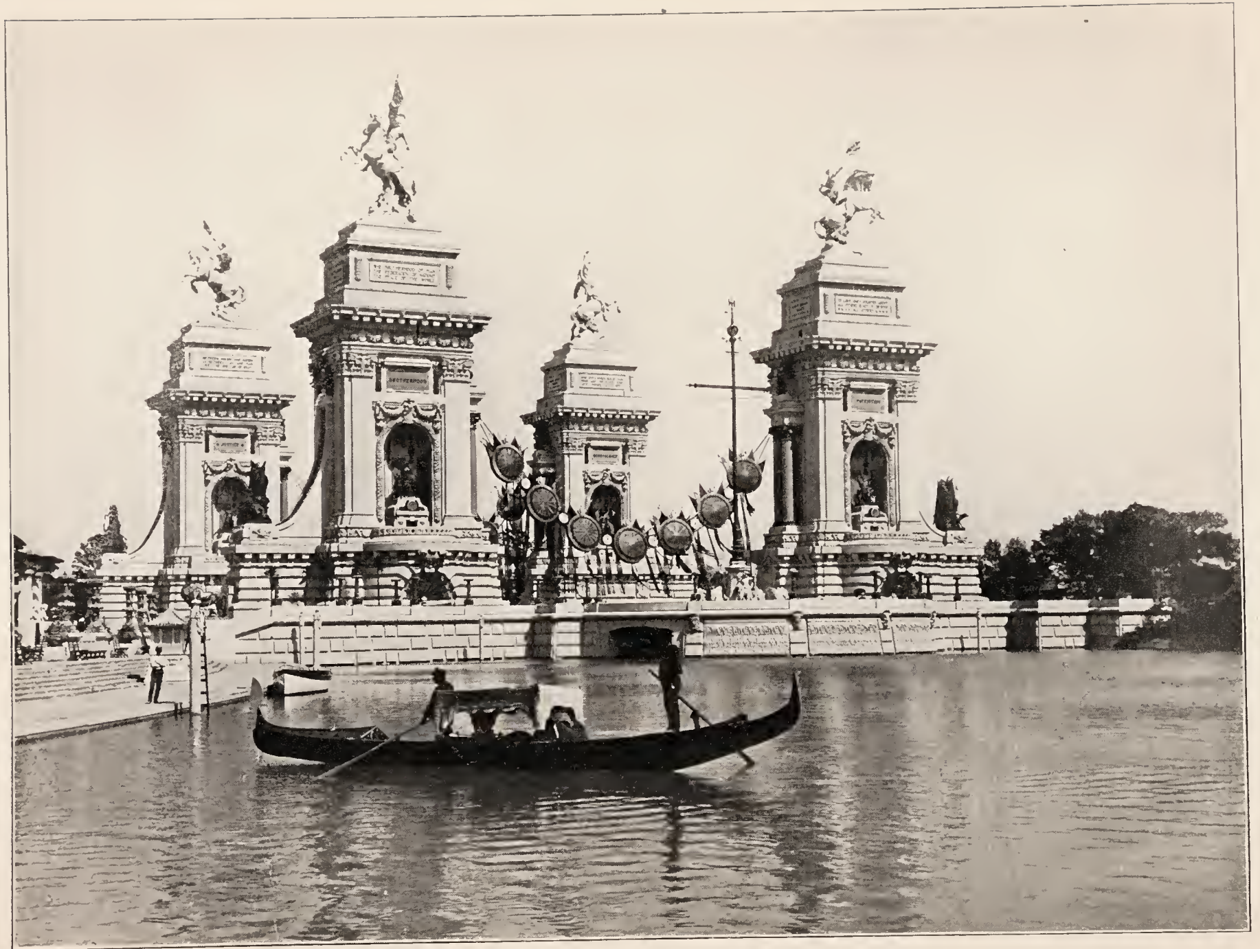
TRIUMPHAL BRIDGE FROM THE MINES BUILDING
