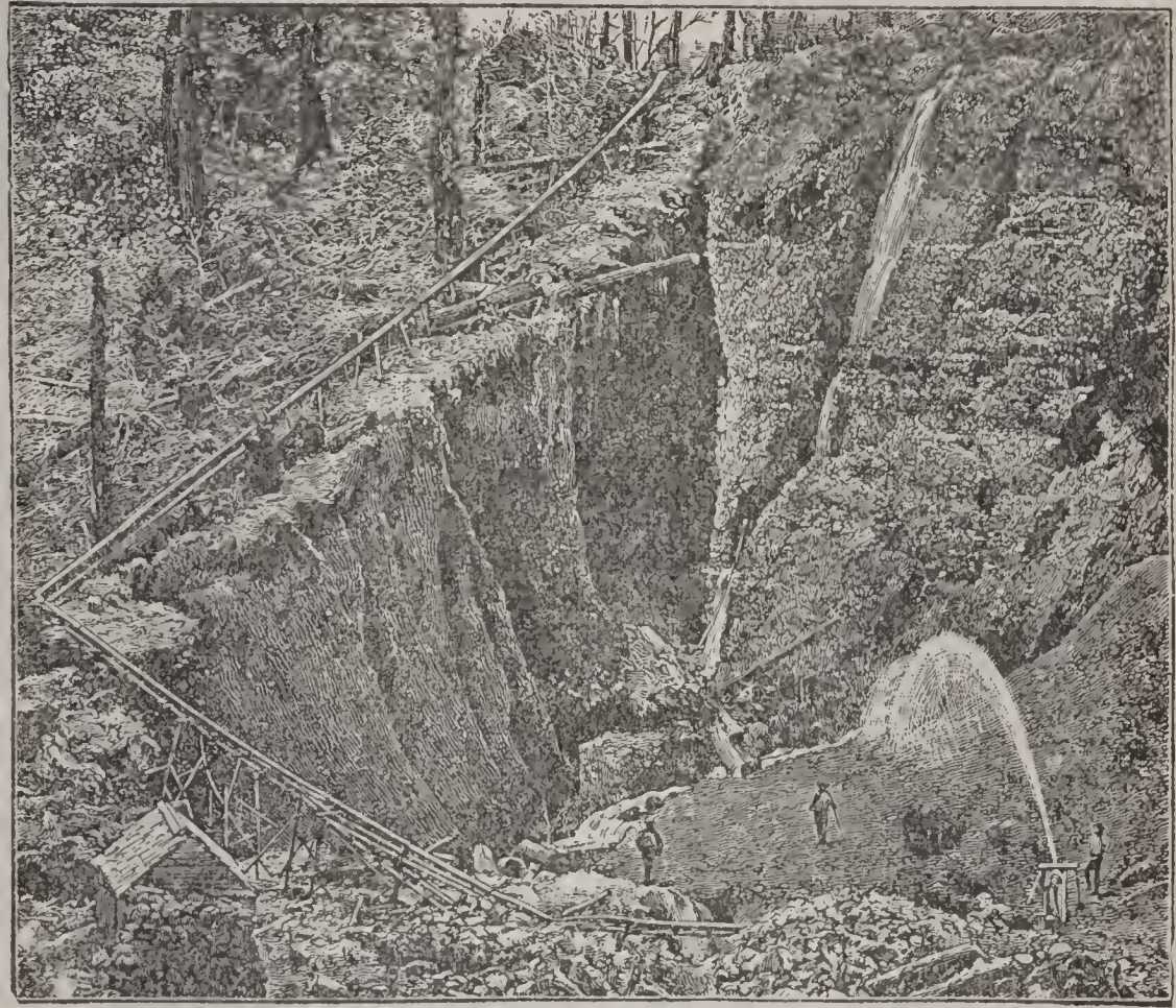
Gold.—Hydraulic Mining, Devil's Creek, Reefton, New Zealand.
