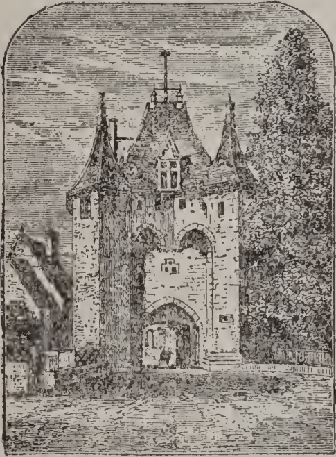
Gate-house at Sens, Villeneuve-sur-Yonne.
