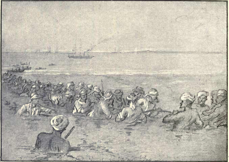
LANDING THE CABLE IN THE MUD AT FĀO
