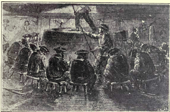
COILING THE CABLE ABOARD
