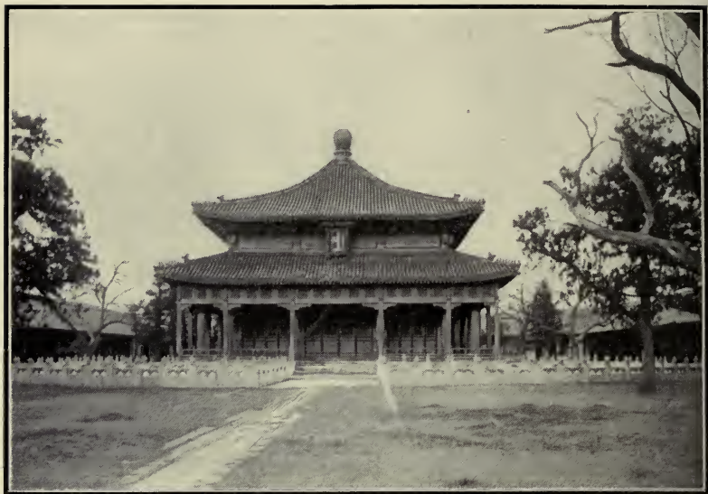
THE IMPERIAL LECTURE ROOM, OLD UNIVERSITY BUILDING
