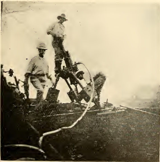
DRILLING AT CULEBRA CUT (1908)
