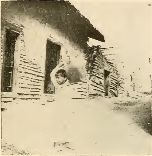
BAMBOO HOUSES AND SAND STREET, PAYTA
