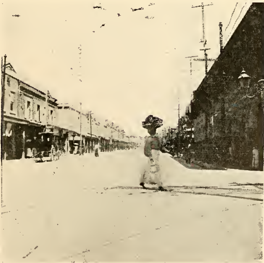
MAIN STREET, KINGSTON, BEFORE EARTHQUAKE
