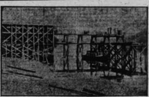
The bunkers in which copper ore is kept ready for loading at one of the mines on Quatsino Sound can be seen at the left. These bunkers are filled by "buckets" which run along an aerial railway from a point thousands of feet up the mountainside where the ore is mined. To the right is the loading wharf, with the Sound in the background.
