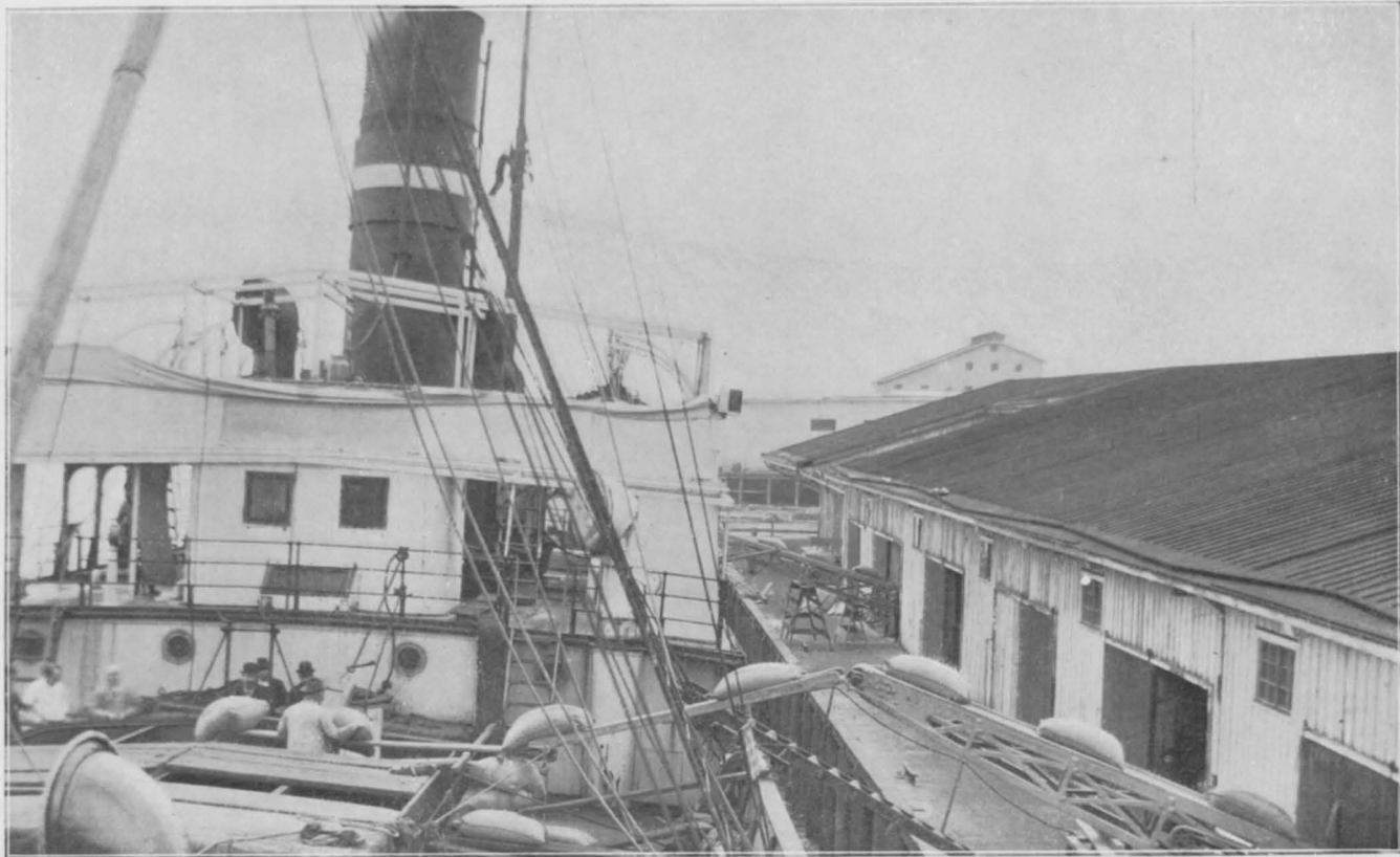
ELECTRICAL CONVEYOR, LOADING 240-POUND SACKS OF WHEAT.
