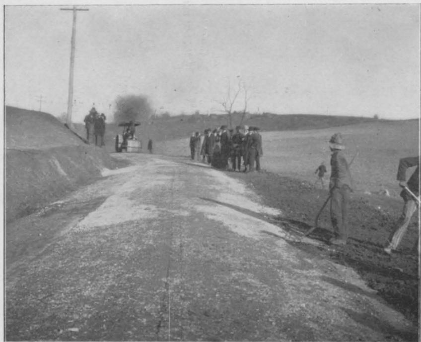
FIG. 2.—OBJECT-LESSON MACADAM ROAD AT GREENEVILLE, TENN.
