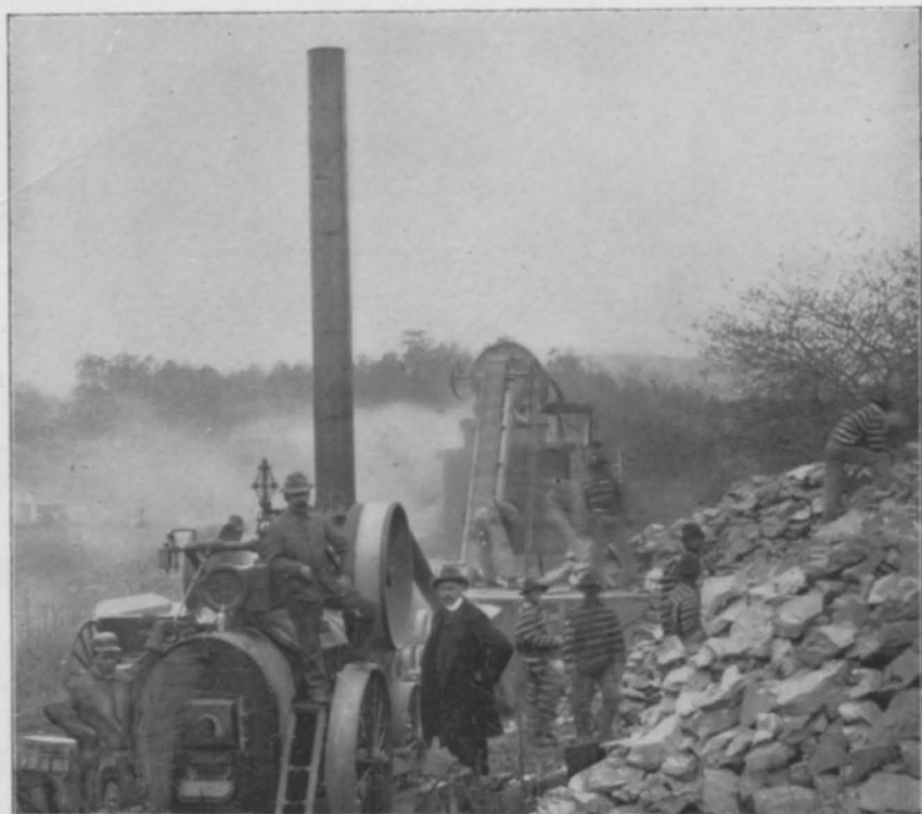
FIG. 1.—UTILIZING CONVICT LABOR IN THE PREPARATION OF ROAD MATERIAL FOR OBJECT-LESSON ROAD AT ASHEVILLE, N. C.
