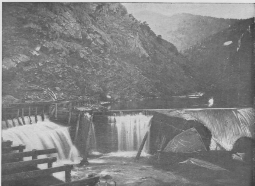
FIG. 1.—DAM AND HEADWORKS OF HANDY DITCH, BIG THOMPSON RIVER, COLORADO.
