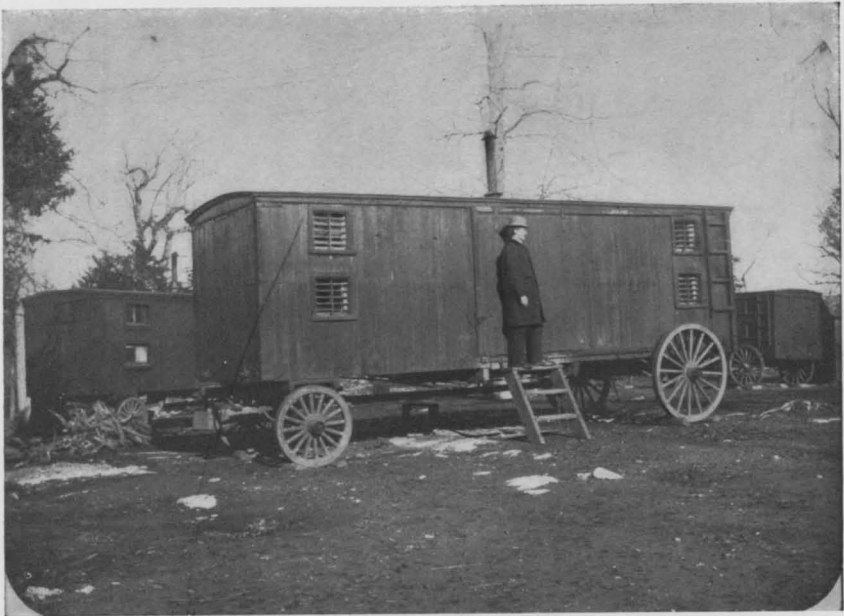
FIG. 1.—PORTABLE CONVICT QUARTERS ON WHEELS, USED FOR THE CONVICT FORCE WORKING ON THE PUBLIC ROADS IN DAVIDSON COUNTY (ABOUT NASHVILLE), TENN.
