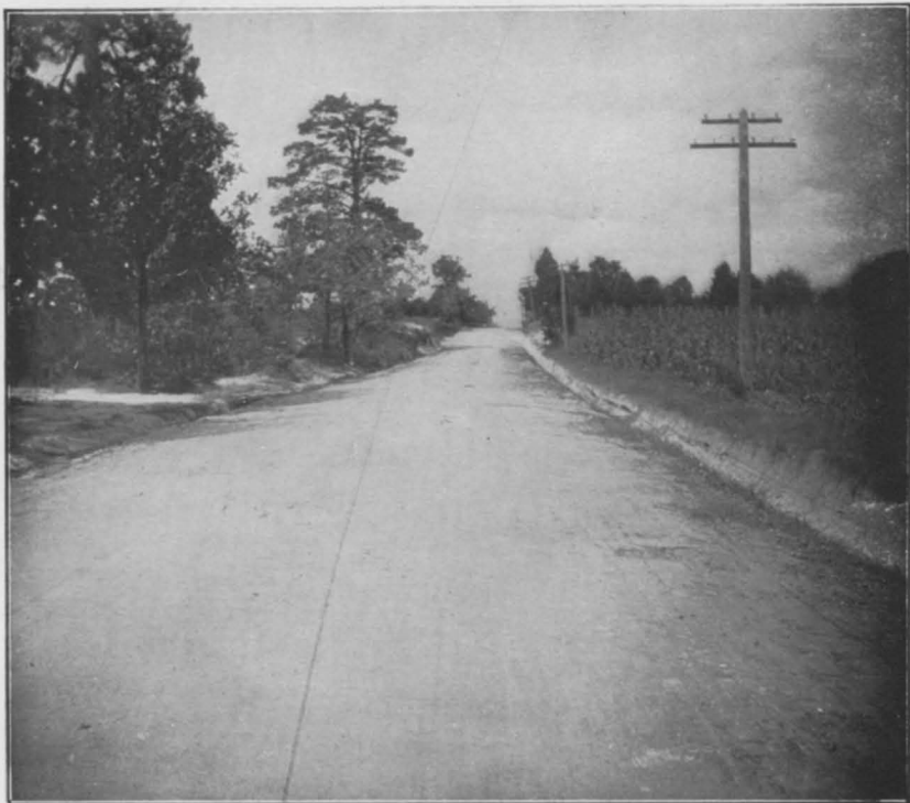
FIG. 2.—A SAND-CLAY ROAD BUILT BY CONVICT LABOR IN RICHLAND COUNTY, S. C.
