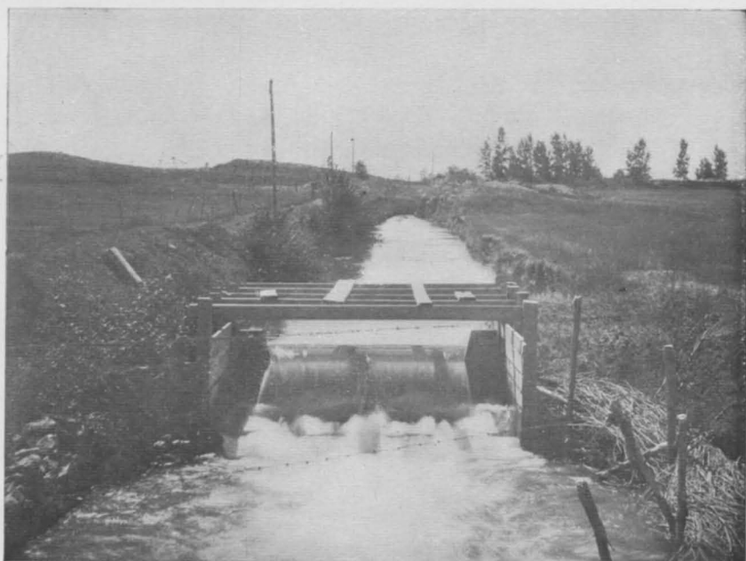
FIG. 2.—WEIR IN OUTLET OF LONE TREE RESERVOIR, COLORADO.
