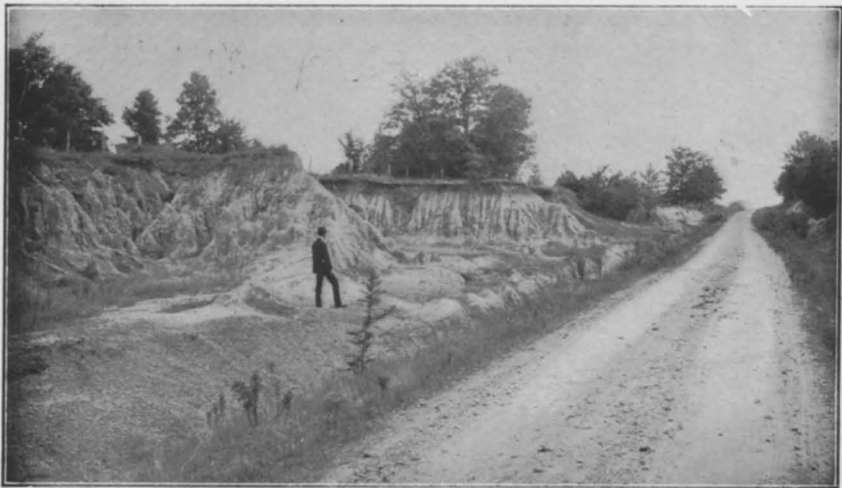
FIG. 2.—GRAVEL ROAD, SHELBY COUNTY, TENN., ABOUT 12 MILES NORTHEAST OF MEMPHIS.
