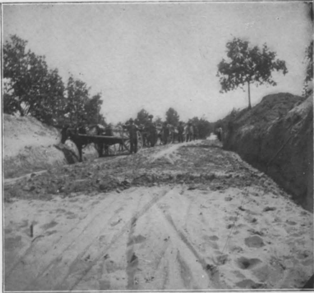
FIG. 1.—HAULING AND PULLING DOWN CLAY ON SAND-HILL ROAD.
