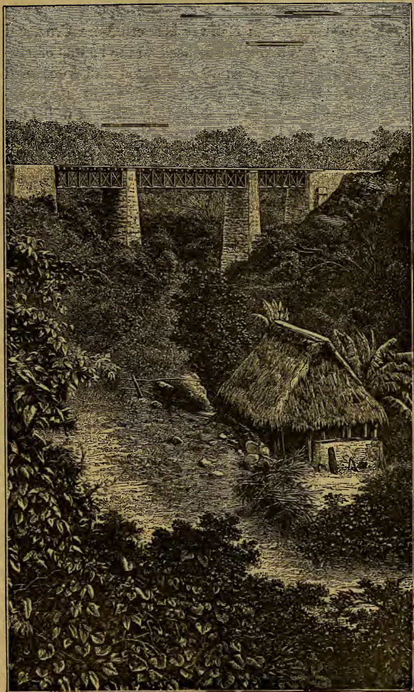
HIGH BRIDGE ON THE MEXICO AND VERA CRUZ RAILWAY.
