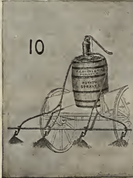
Fig. 10. FOUR ROW SPRAYING ATTACHMENT. Cut shows this attachment as used on an ordinary wagon. We furnish this attachment complete, less barrel, pump and wagon. . . . . Our net price 10.00
