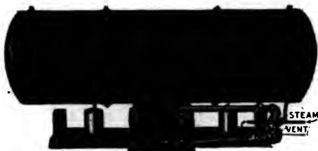
The Farnsworth Duplex Boiler Feeder—rear view of 3-inch machine, showing steam and vent connections, controlling alternate chambers. This machine is really two traps in one—while one side is discharging the condensation under pressure, the other side is filling. It works with a continuous, automatic flow.
