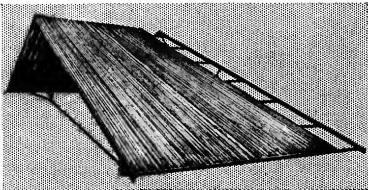
Taking as a basis the stress and strain of wind and snow, we built our main truss to stand strains and stresses largely in excess of its needs. To make sure it would stand that excess, the roof was loaded down with a dead weight of iron bars. Not till then did we decide to use that truss in our Standard Iron Frame Construction.
