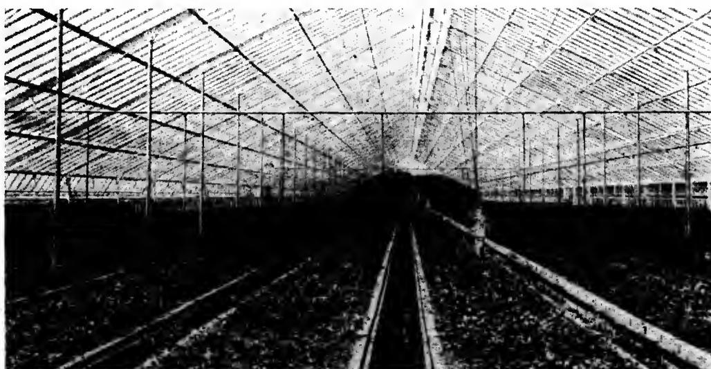
This house of A. S. Burns at Spring Valley, N. Y., is 69 ft. 6 in. wide and 400 ft. long. We consider it one of our model widths and construction.
