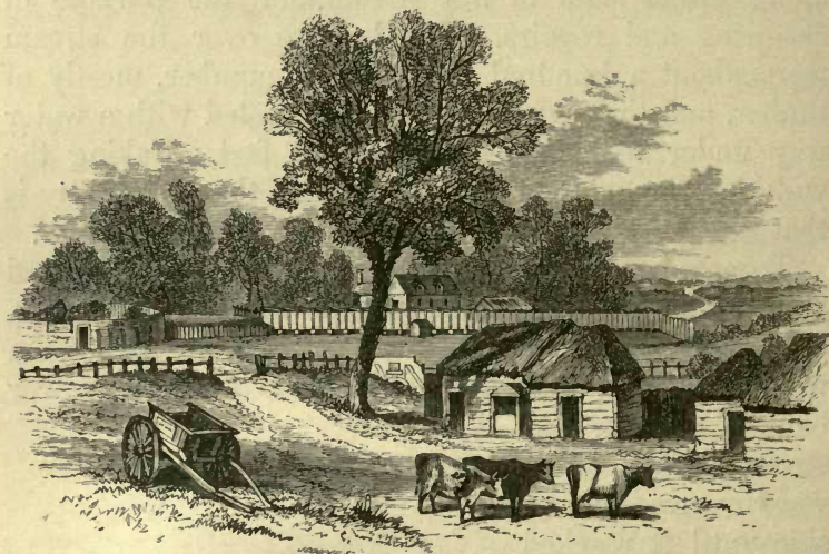
THE BOARDED RIVER FORMERLY AT BUSH HILL.
