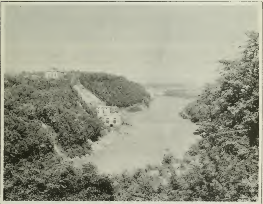
QUEENSTON-CHIPPAWA POWER DEVELOPMENT Power house in lower Niagara gorge, looking north towards Queenston from University Point on the United States side of the Niagara river
