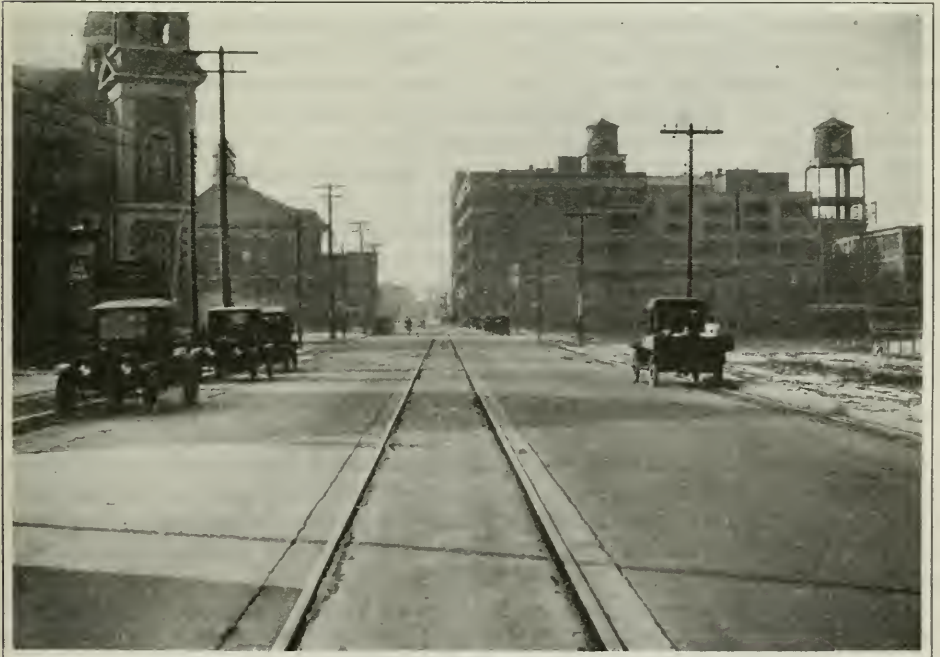
ESSEX DISTRICT RAILWAYS Sandwich Street, Ford City, after rehabilitation
