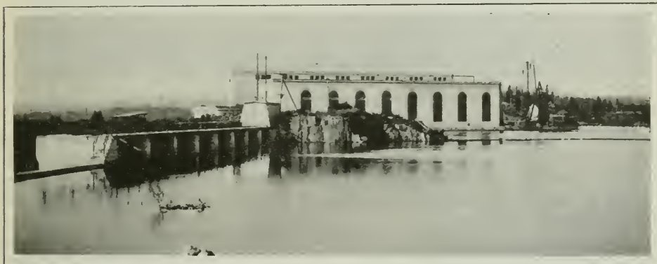
NIPIGON POWER DEVELOPMENT Dam and headworks from upstream side of development
