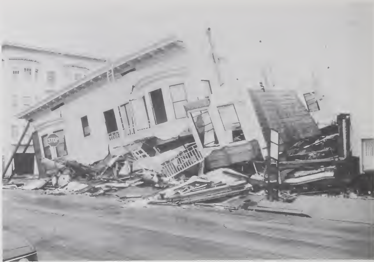
Figure 4.2.8 Four-story building which suffered total collapse of its lower stories (location #3).
