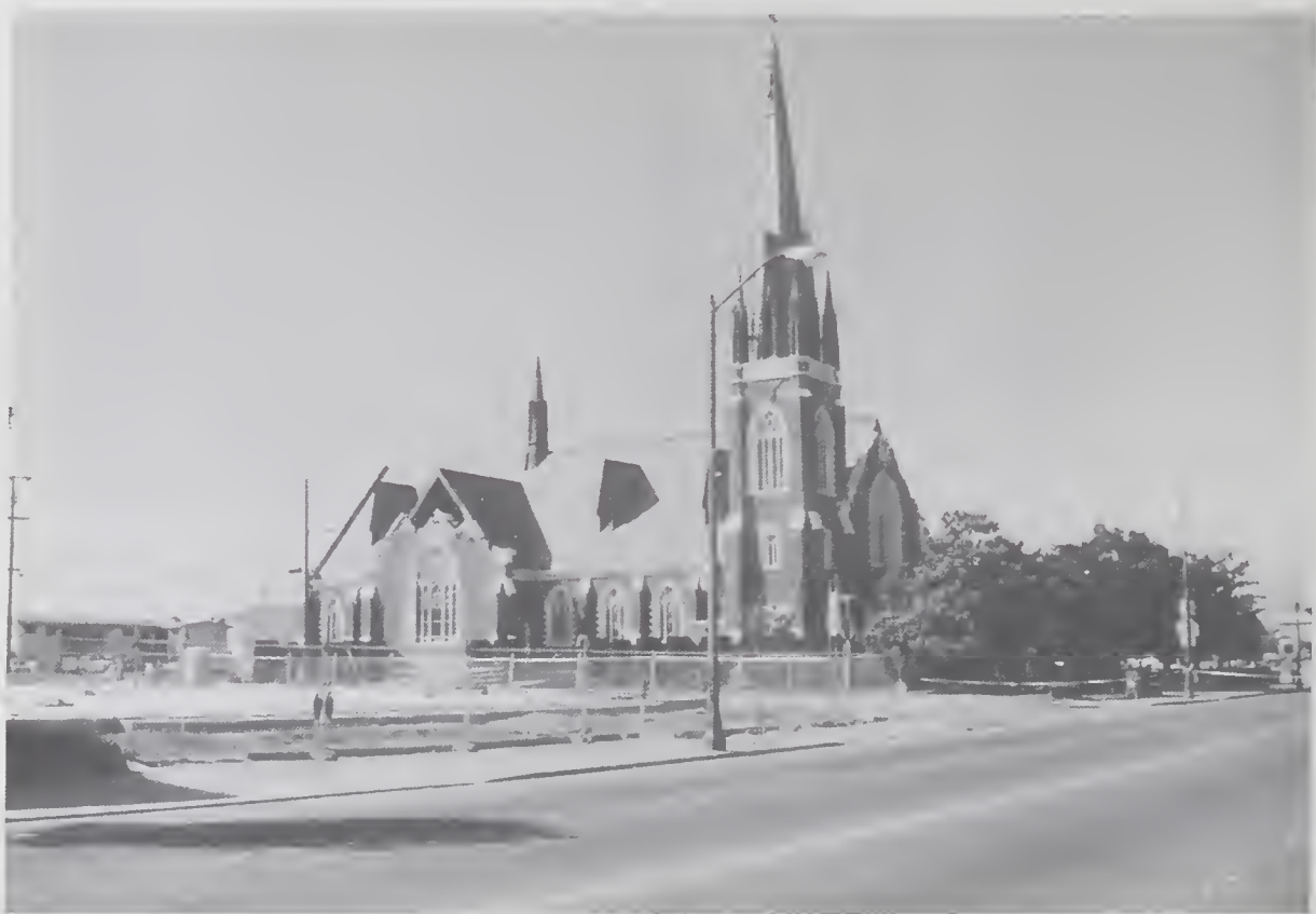
Figure 4.4.6 St. Patrick's Church in Watsonville was severely damaged.
