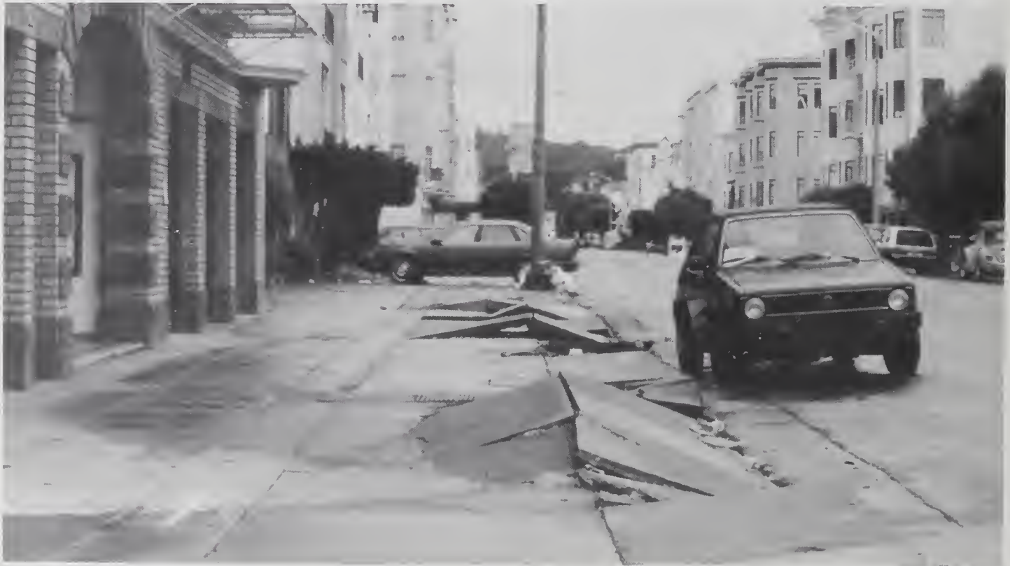
Figure 3.3.4 Typical liquefaction damage in the Marina District of San Francisco.
