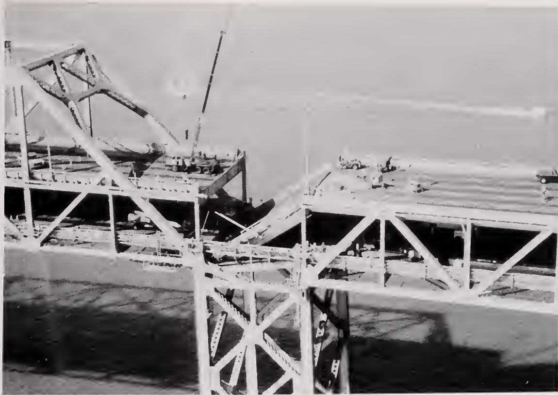
Figure 5.7.4 Aerial photo looking north at Pier E-9 on October 19, 1989 showing the collapsed upper and lower 50 foot deck spans.
