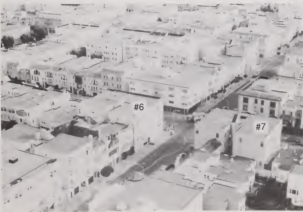
Figure 4.2.21 Aerial view (#4) of the buildings shown in figures 4.2.12 and 4.2.20.
