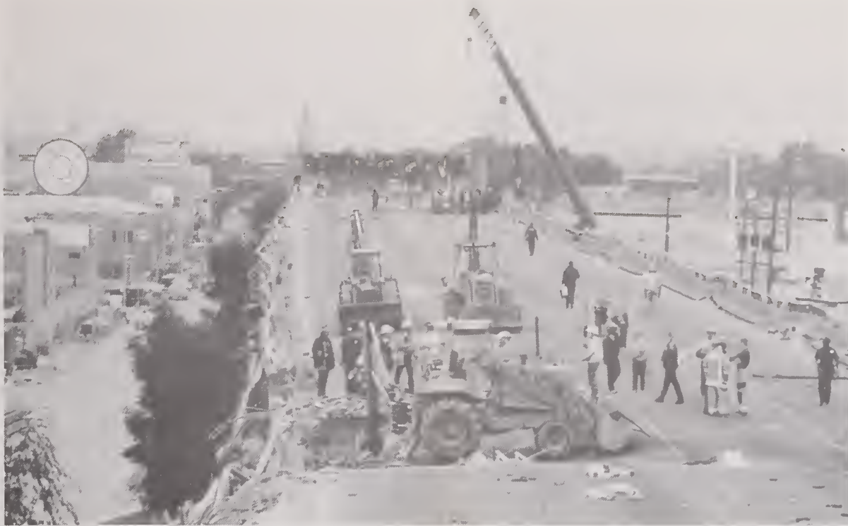
Figure 5.6.24 View of the upper deck of Cypress Structure looking north of Bent 80. This photo illustrates the negligible lateral displacement of the upper deck relative to the lower deck during the collapse.
