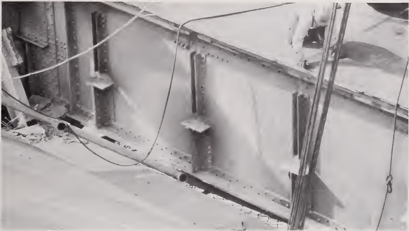
Figure 5.7.7 Close-up of the western girder seats for the lower road deck at Pier E-9. Lack of significant damage to these seats, and to those supporting the upper road deck, indicates that both upper and lower segments moved eastward by an amount sufficient to permit both to slide off the western seats and drop simultaneously.
