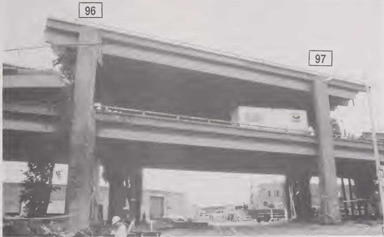
Figure 5.6.36 View looking west towards Bents 96 and 97 which supported the only segment of the upper deck to remain standing between Bents 62 and 113.
