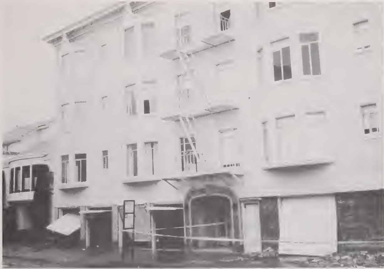
Figure 4.2.10 Example of four-story building with multiple garages in the first story (location #4).
