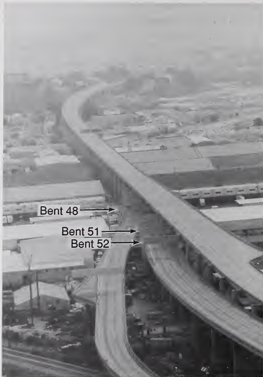
Figure 5.9.2 Aerial view of I-280 south of Army St., note the transition from a two-level elevated structure to a single-level, divided structure (view is looking south).
