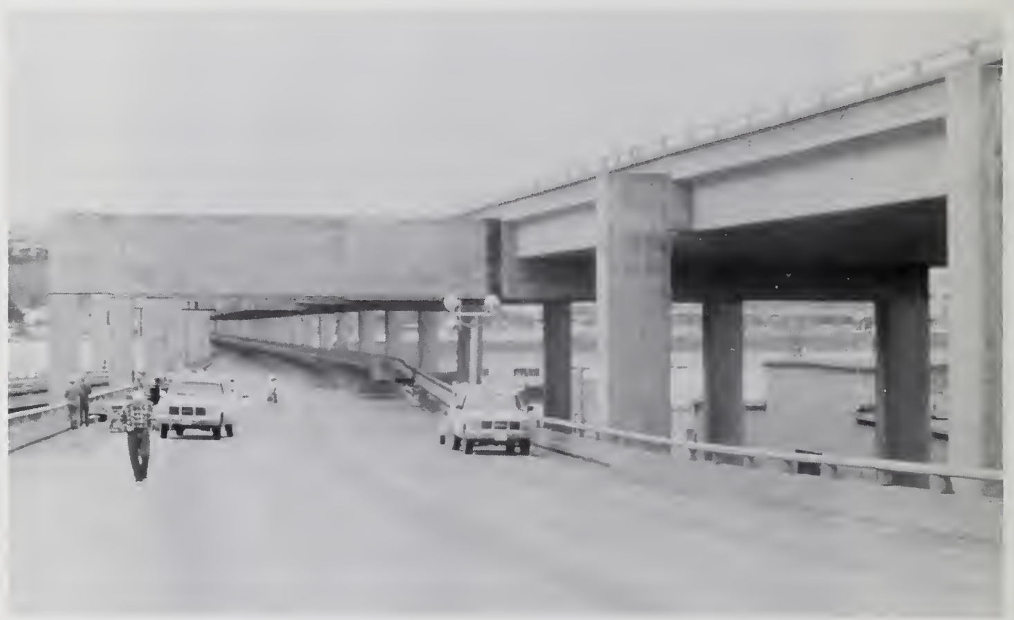
Figure 5.9.6 View looking south on I-280 showing the upper girder of Bent 52.
