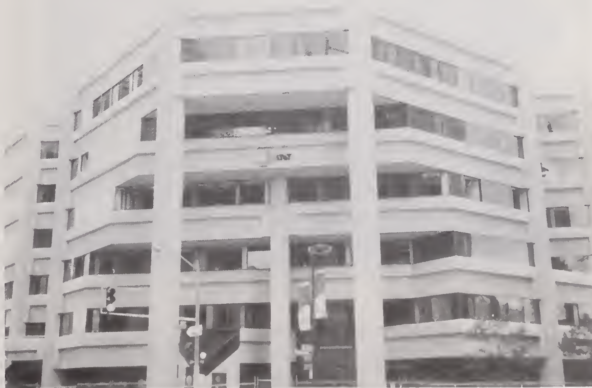
Figure 4.3.7 Trans Pacific Centre Building which suffered extensive damage due to ruptured water pipes, broken windows, and fallen ceiling tile (location #4).
