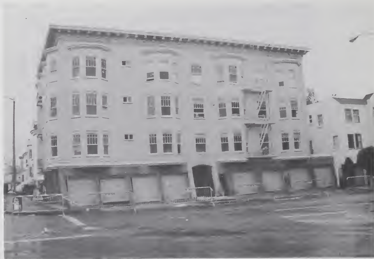
Figure 4.2.9 Example of four-story building with multiple garages in the first story (location #1).
