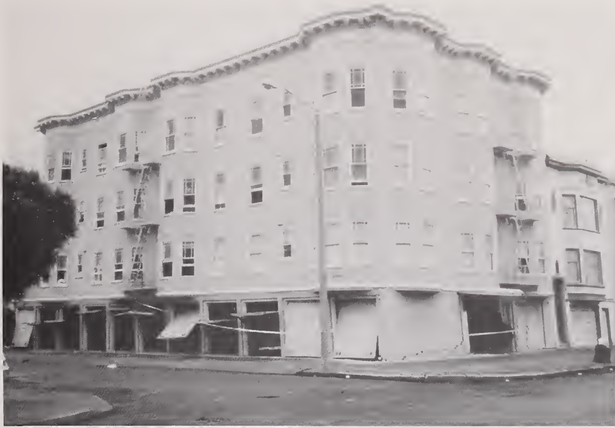
Figure 4.2.14 Example of four-story building with multiple garages in the first story (location #13).
