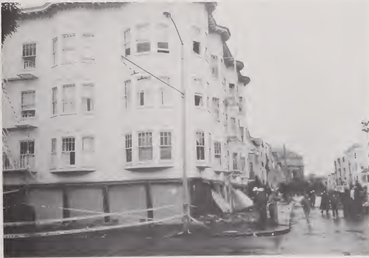
Figure 4.2.11 Example of four-story building with multiple garages in the first story (location #5).
