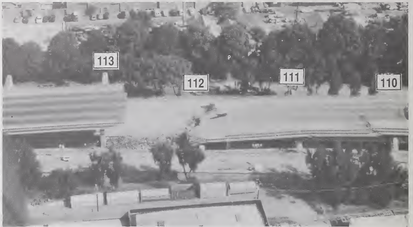
Figure 5.6.10 Aerial photo looking east to the northern limit of the collapsed portion of Cypress Structure between Bents 110-113.
