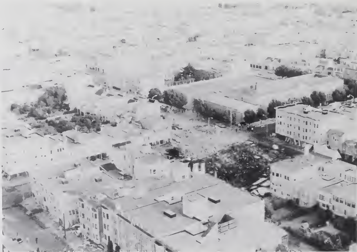
Figure 4.2.5 Aerial view (#3) of portion of the Marina District which suffered extensive damage; dark zone is location of the fire.
