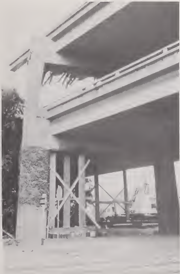
Figure 5.6.36 View looking west towards Bents 96 and 97 which supported the only segment of the upper deck to remain standing between Bents 62 and 113.
