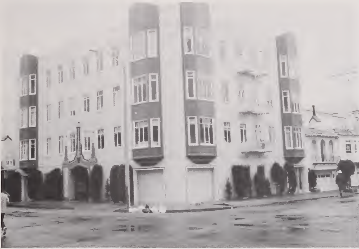
Figure 4.2.20 An undamaged four-story building on the corner of Broderick and Beach Streets (location #7).
