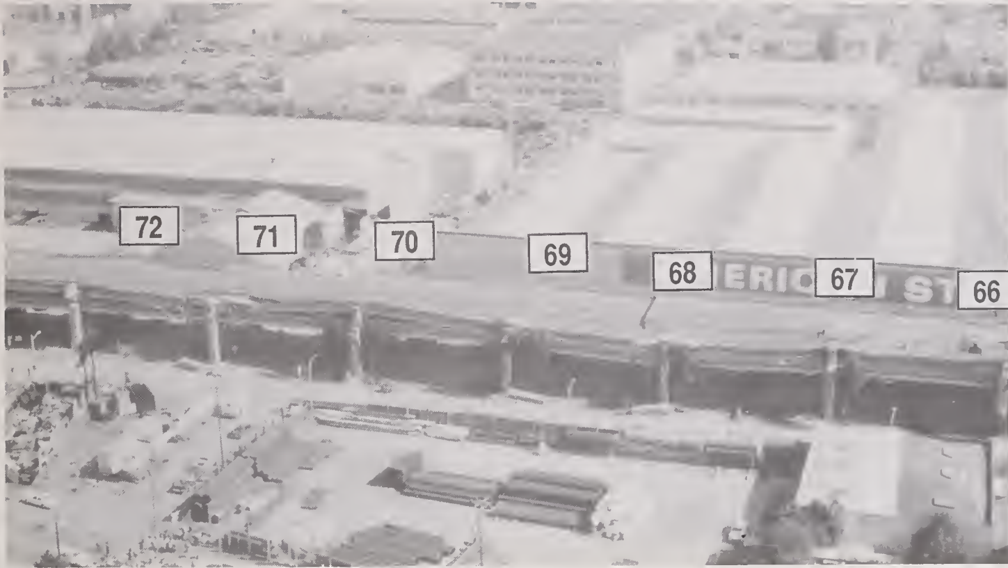
Figure 5.6.20 Aerial photo looking east to the collapsed portion of Cypress Structure between Bents 66-72.
