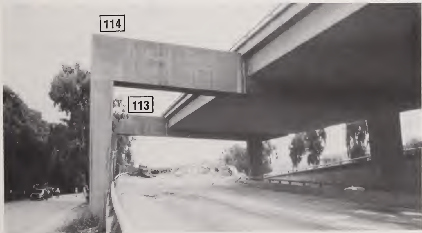
Figure 5.6.41 View looking south along the east side of Cypress Structure from Bent 115. The northern limit of the collapse extended to within six feet of Bent 113.
