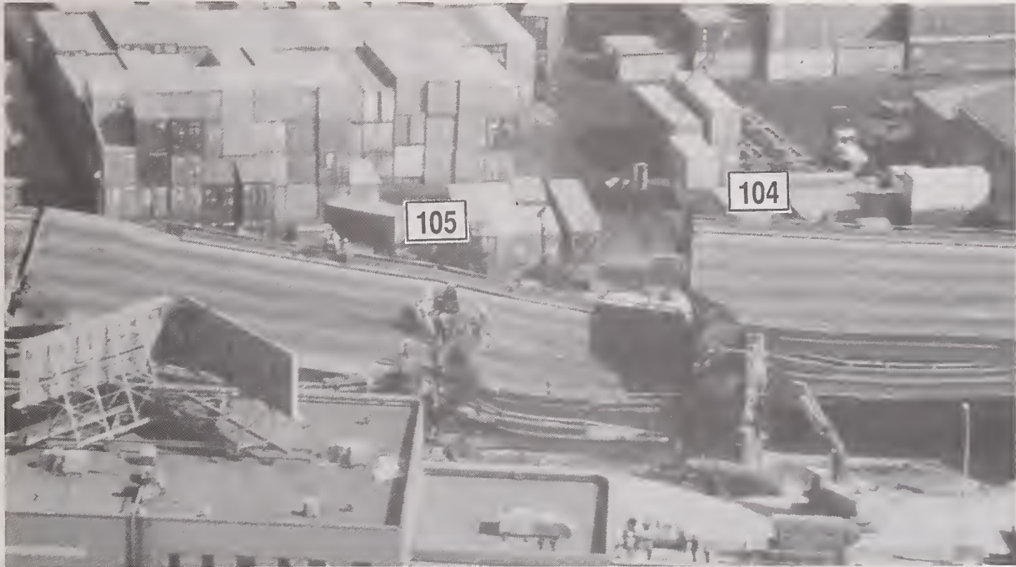
Figure 5.6.12 Aerial photo looking east to the collapsed portion of Cypress Structure between Bents 104-106.
