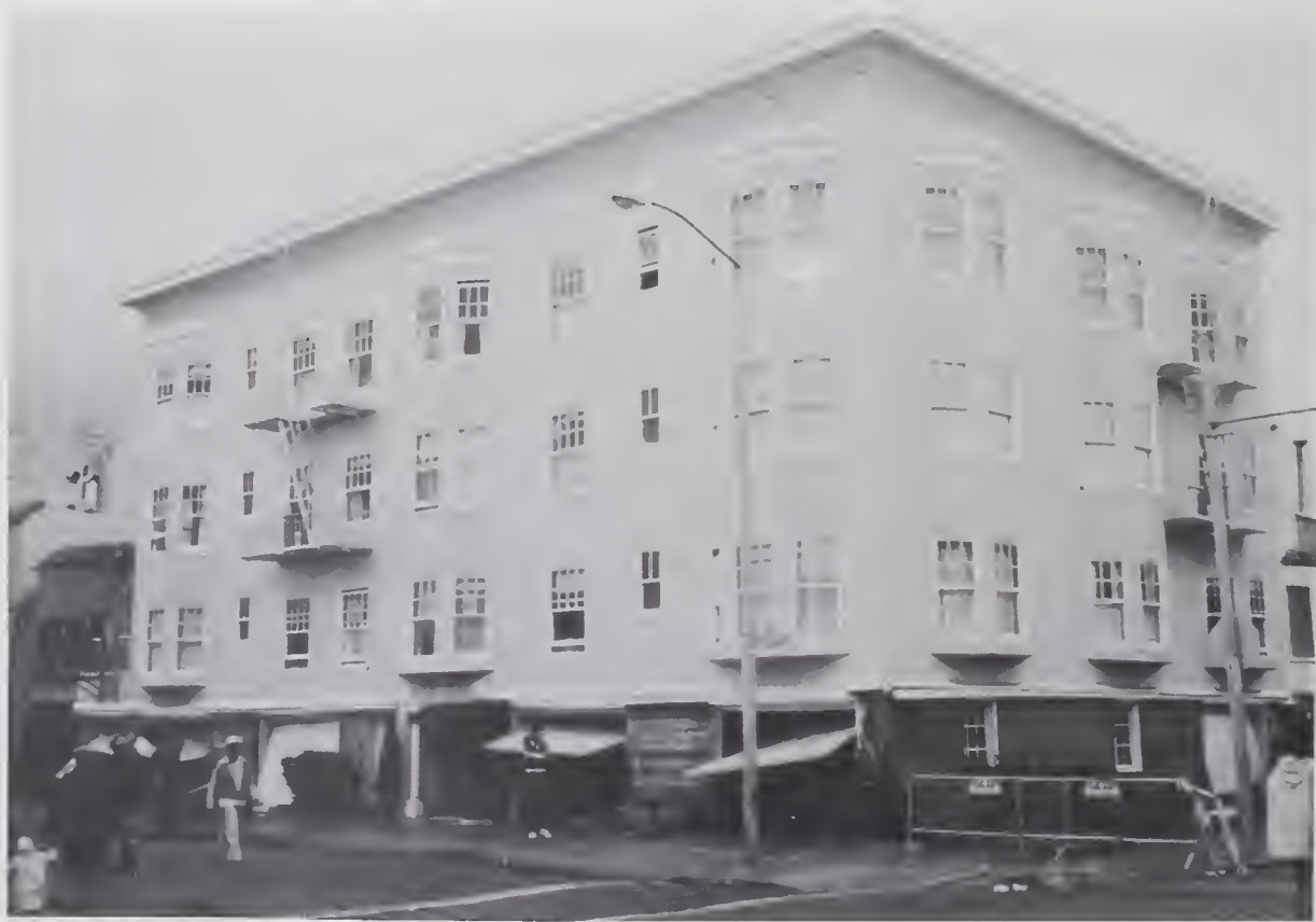
Figure 4.2.13 Example of four-story building with multiple garages in the first story (location #9).
