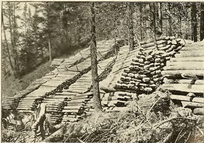
FIG. 2.—TIE PILES AT THE FLUME.
