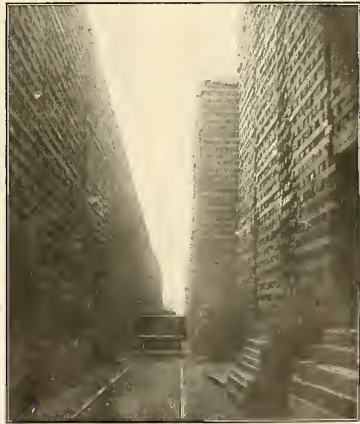
FIG. 4.—ANOTHER VIEW OF FIG. 2. PILING PINE ON THE GREAT WESTERN RAILWAY, ENGLAND.
