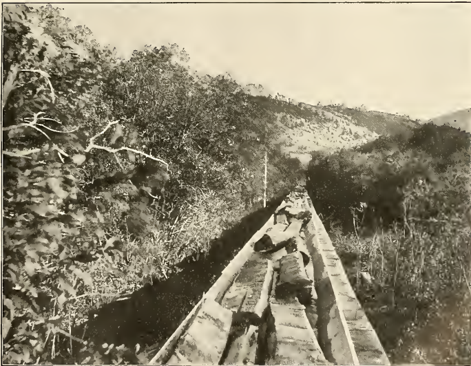
FIG. 2.—ANOTHER VIEW OF FLUME.
