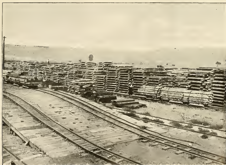
FIG. 2.—TIE YARD, SHERIDAN, WYO., SEPTEMBER, 1902—OPEN PILES.
