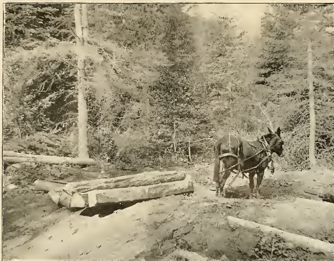
FIG. 1.—DRAGGING TIES TO THE FLUME.
