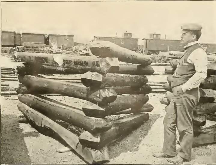
FIG. 1.—TRIANGULAR TIE PILES.
