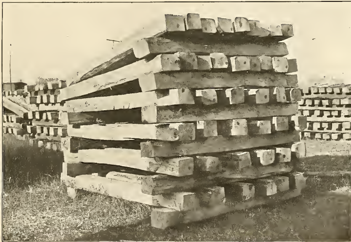
FIG. 2.—ANOTHER METHOD OF ROOF BUILDING.
