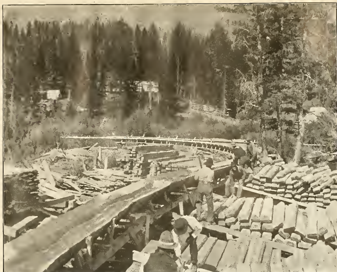
FIG. 1.—THROWING TIES INTO THE FLUME.
