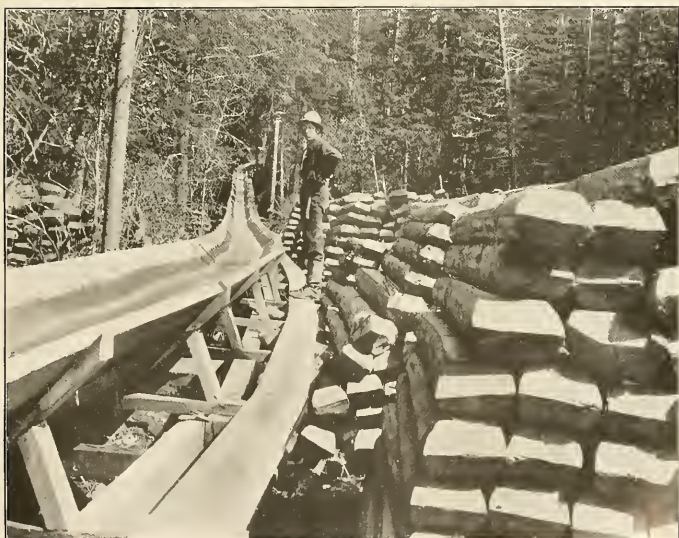
FIG. 2.—TIES READY FOR THE FLUME.
