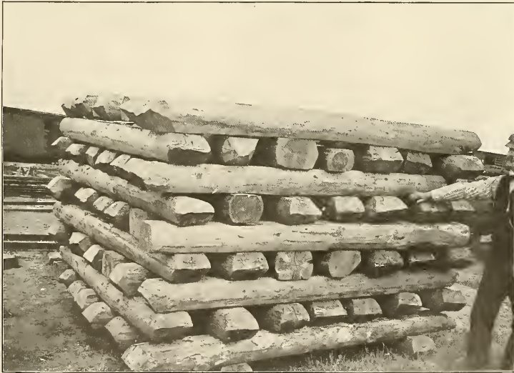
FIG. 2.—LOGGEPOLK PINE—HALF-OPEN PILE.
