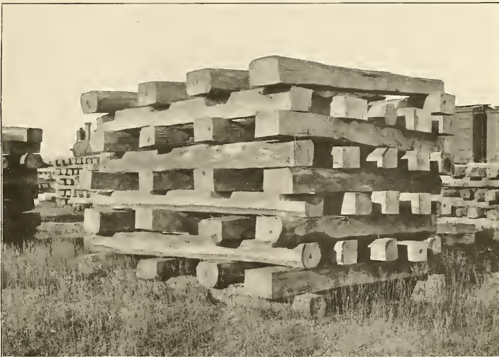
FIG. 2.—ANOTHER OPEN-CRIB PILE.
