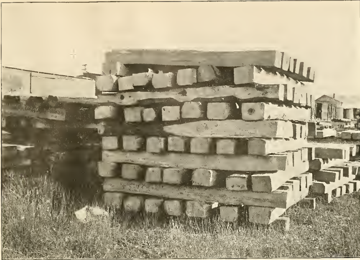
FIG. 1.—OAK PILES, SHOWING METHOD OF BUILDING A ROOF.
