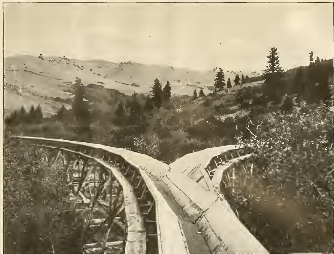
FIG. 1.—END OF FLUME AT RAILROAD TRACK.
