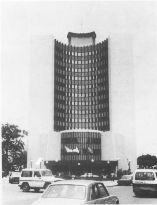
The Hydro Congo building.
