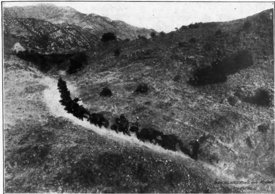
PACK TRAIN WITH 2500 FT. OF \frac{3}{4} -IN. STEEL ROPE FOR THE PALMAREJO MINE, CHIHUAHUA
