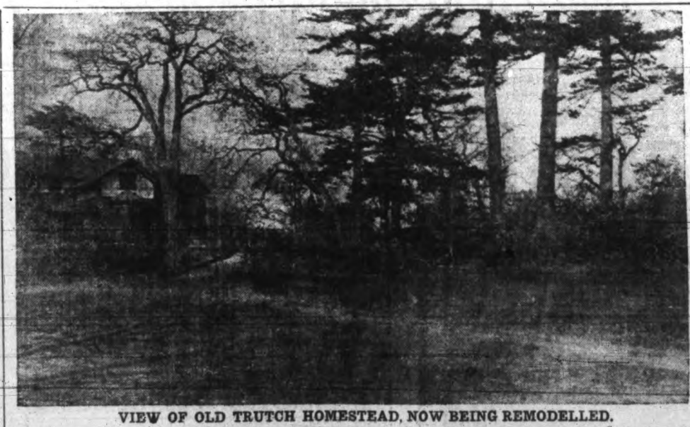
VIEW OF OLD TRUTCH HOMESTEAD, NOW BEING REMODELLED.
