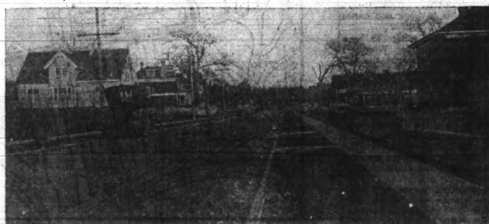
A NEWLY BUILT PORTION OF COLLINSON STREET.
