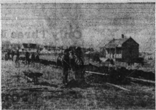
LAYING NEW WATER MAINS ON CHAPMAN STREET
