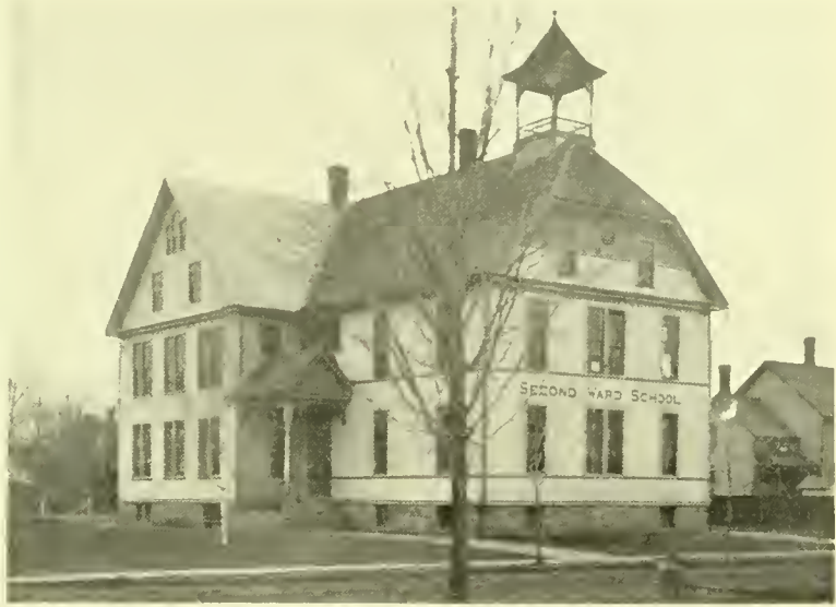
Butler, Photo. SCHERMERHORN STREET SCHOOL.
