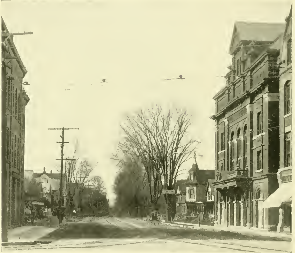
Photo by Hyatt. GROTON AVENUE, WEST FROM MAIN STREET. [Opera House.]
