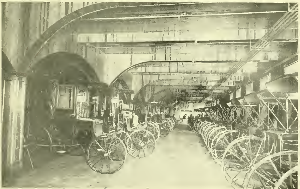
Hyatt, Photo. REPOSITORY CORTLAND WAGON CO., LOOKING WEST ON NORTH SIDE.
