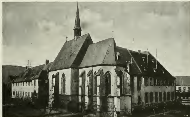
THE HOSPITAL AT CUES, GERMANY
