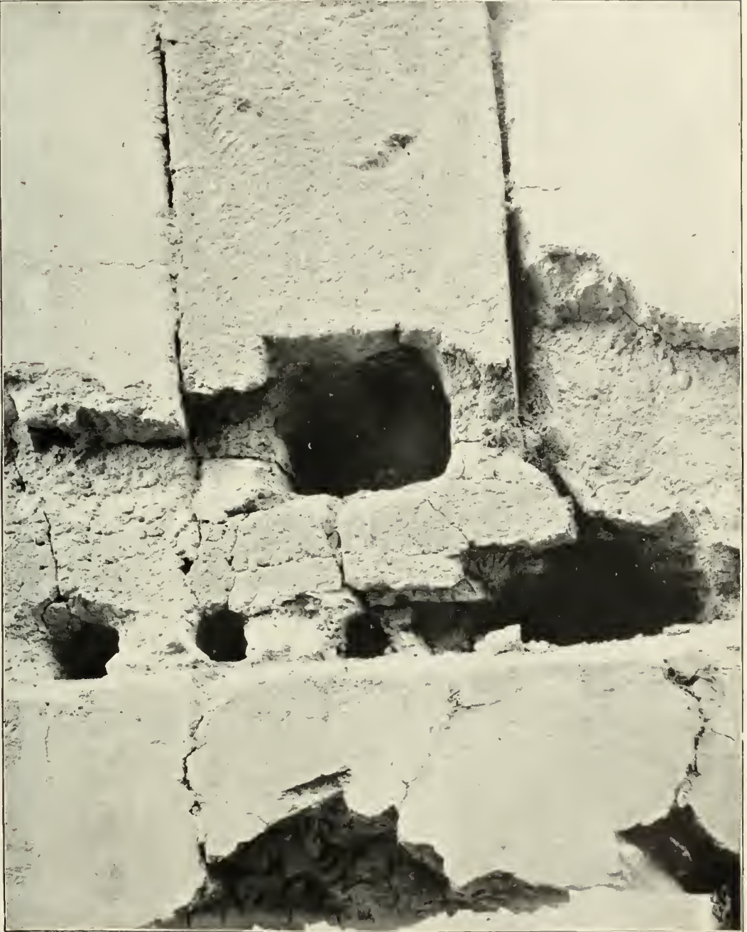
BLOCKED OPENING IN WEST WALL.
