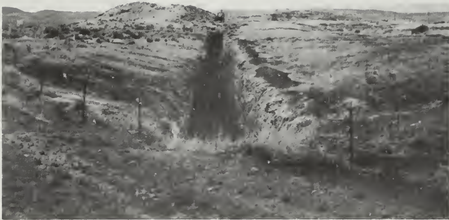
Figure 44. Miners excavated trenches to reach the gilsonite veins, which trend to the southeast north of the White River. Many trenches are hundreds of feet deep.
