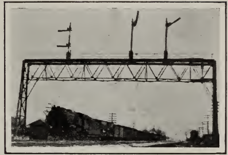
SIGNAL BRIDGE NEAR SUMMIT
