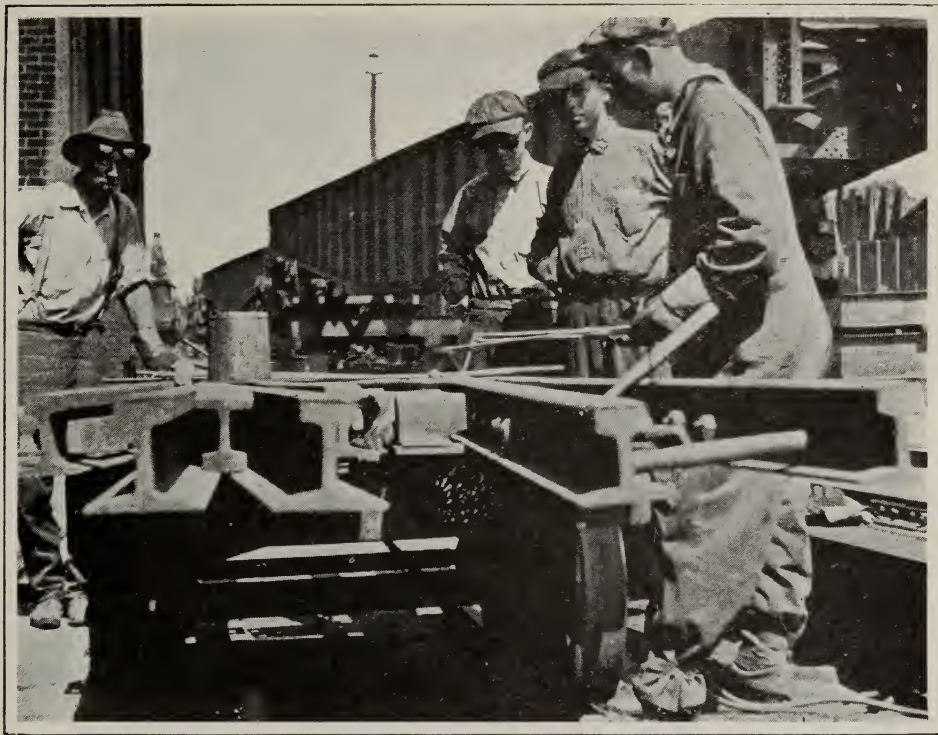
CREW REFACING FROGS AT MARTINSBURG SHOPS
