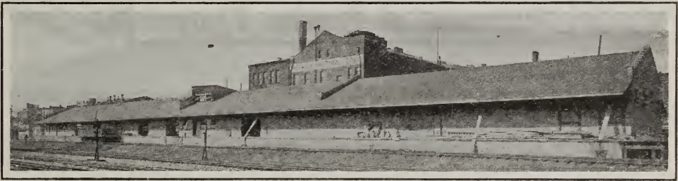
Fine New Freight House at Braddock, Pa., Viewed From South Side
