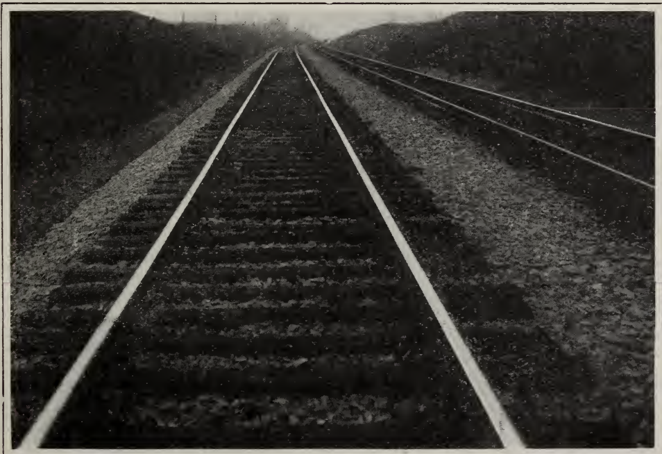
Standard Track West of Charlestown Station—New Castle Division
