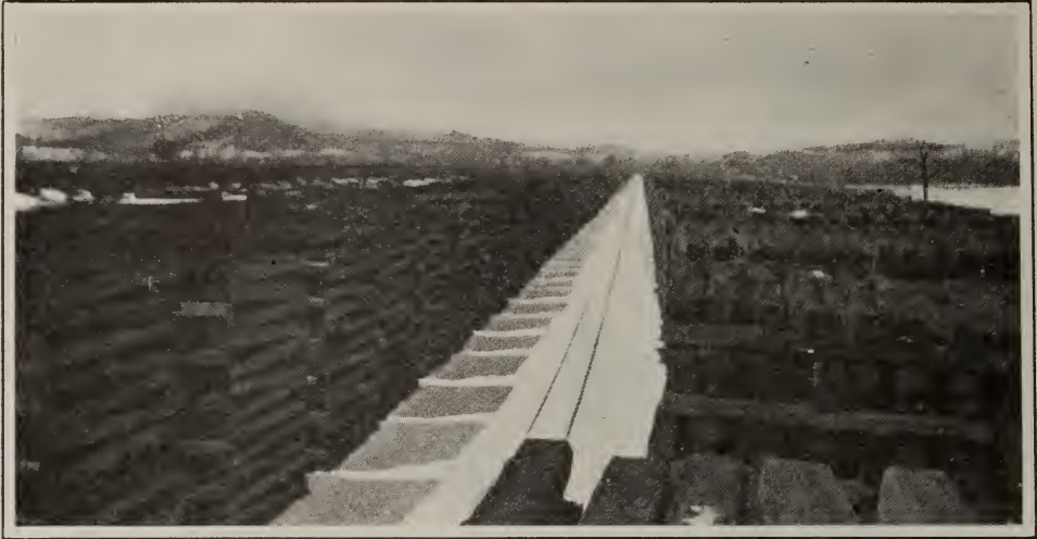
TRACK No. 7, TIMBER PRESERVATION PLANT, GREEN SPRING, W. VA.
