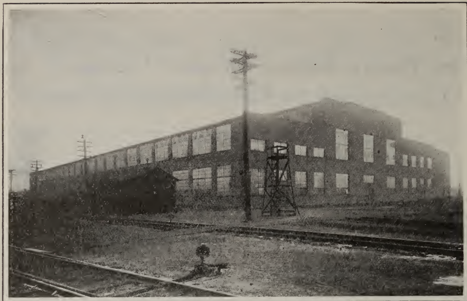
South Cumberland Shops—View from Northwest, showing North and West Walls of the Shop
