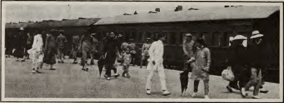
SCENE AT RAILWAY STATION AT CHIN WANG TAO
