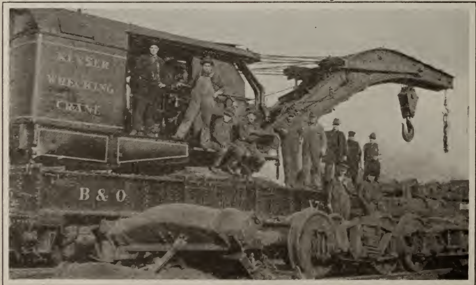
KEYSER WRECKING CREW
