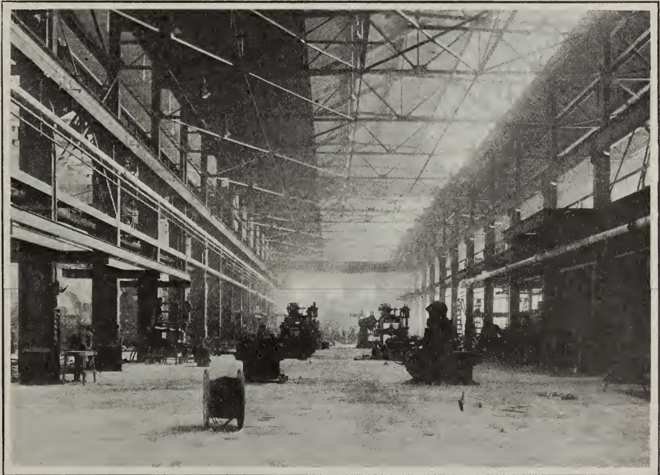
South Cumberland Shops—View taken from the West End of the Machine Shop
