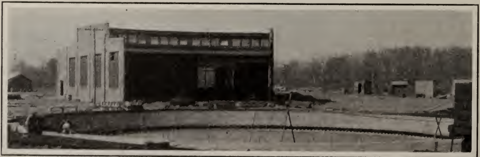
Engine House and Turntable Pit at Elsmere Junction, Del.
