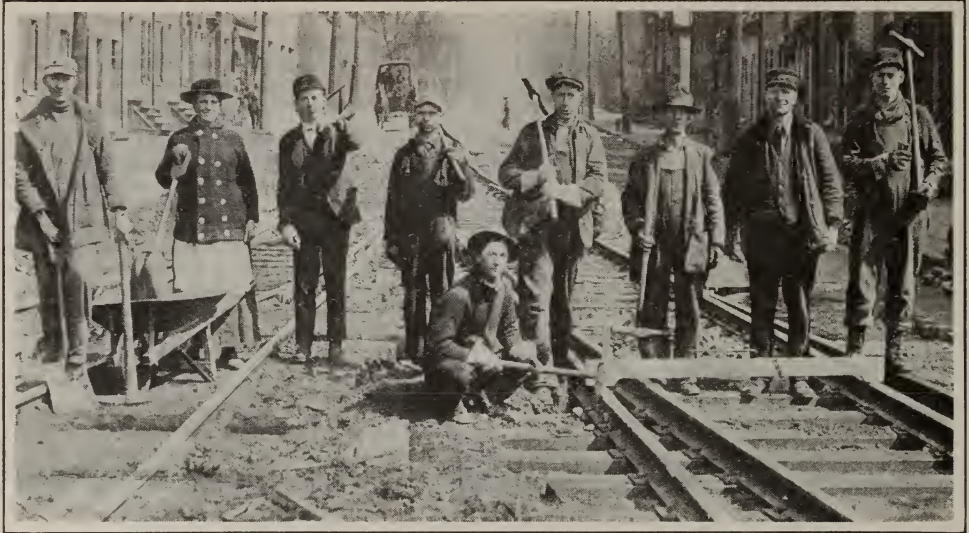
TRACK FOREMAN W. M. LEMLEY (SECOND FROM RIGHT) AND GANG
