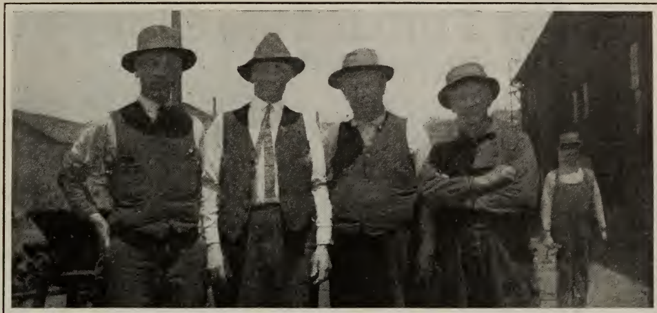
BOILER SHOP FORCE AT GLENWOOD SHOPS
