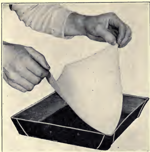
Illustration No. 52 Sensitizing the Paper—Lowering onto the Bath See Paragraph No. 370
