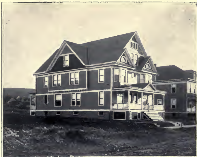
Illustration No. 18 Light Building Properly Photographed See Paragraph No. 109
