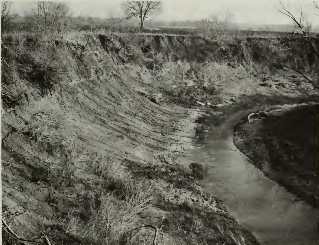
Active streambank erosion in lower reaches of mainstem of Elm Creek is destroying cropland.
