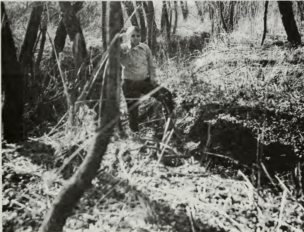
This tree-lined channel on North Elm Creek is almost completely filled with sediment. This channel is being abandoned through new channel formation processes or valley trenching on open areas of the flood plain.
