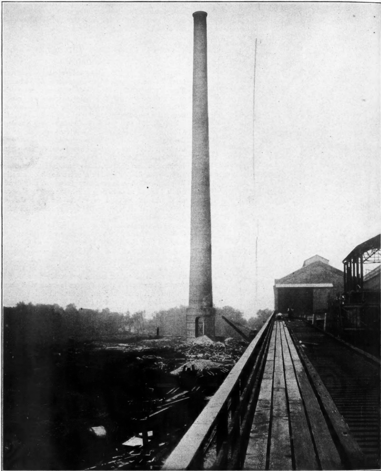
ONE OF TWO 350-FT. CONCRETE CHIMNEYS AT INTERNATIONAL NICKEL CO.'S REFINERY AT PORT COLBORNE These are the highest reinforced-concrete chimneys in North America. They are 350 ft. high, 12 ft. inside diameter at the top and 29 ft. 4 in. outside diameter at the base. Five reinforced-concrete chimneys were built at the Port Colborne refinery by the General Concrete Construction Co. of New York and Chicago. The chimneys were built of a 1:2½:3 mix poured in the special steel forms shown on the opposite page. These forms are adjustable to the taper of the chimney.
