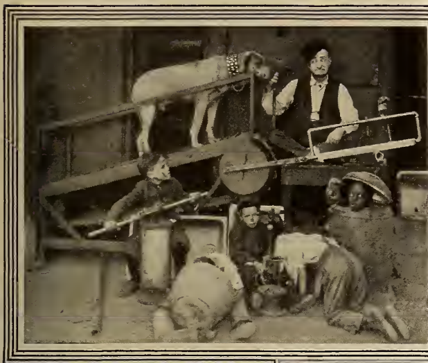
1. Reilly's dog-power saw at work on a piece of pipe. One of Reilly's busy days.
