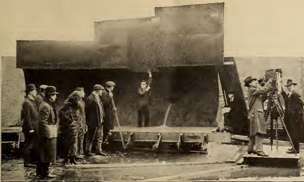
You would never guess what this was unless we told you. It is a scene in a deep, cavernous, horrid sewer, 'way under ground, but for purposes of clear photography, the movie folks built it on a roof, which is where you see it.
