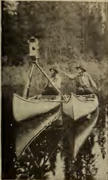
Two guides paddle the canoes. Two legs of tripod in one canoe, one in the other.
