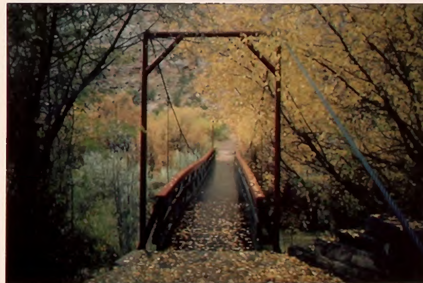
Bridge Across Calf Creek (photo by BLM)
