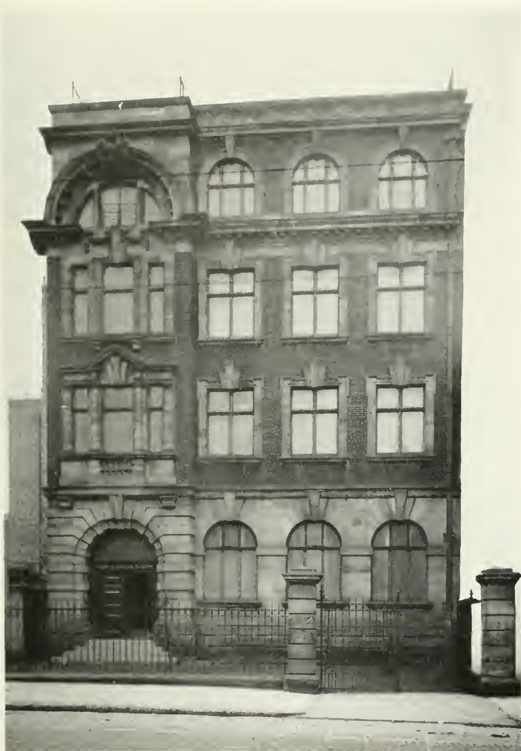
FRONTAGE OF THIRD LABORATORY OF SCHOOL
