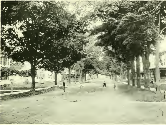
A. Johnson, Photo. CORTLAND STREET, looking north from the bridge
