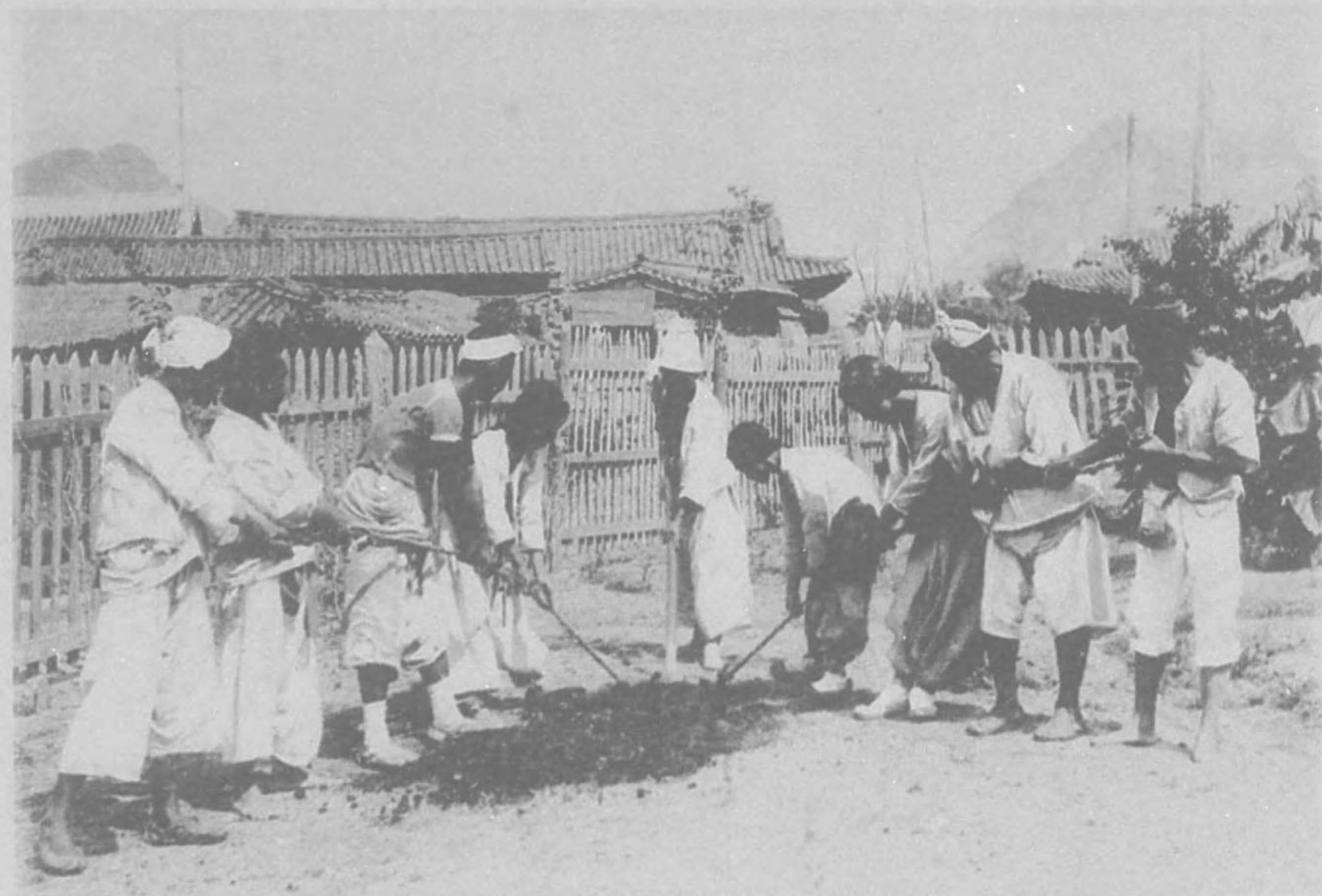
掘 土 Coolies digging ground.
