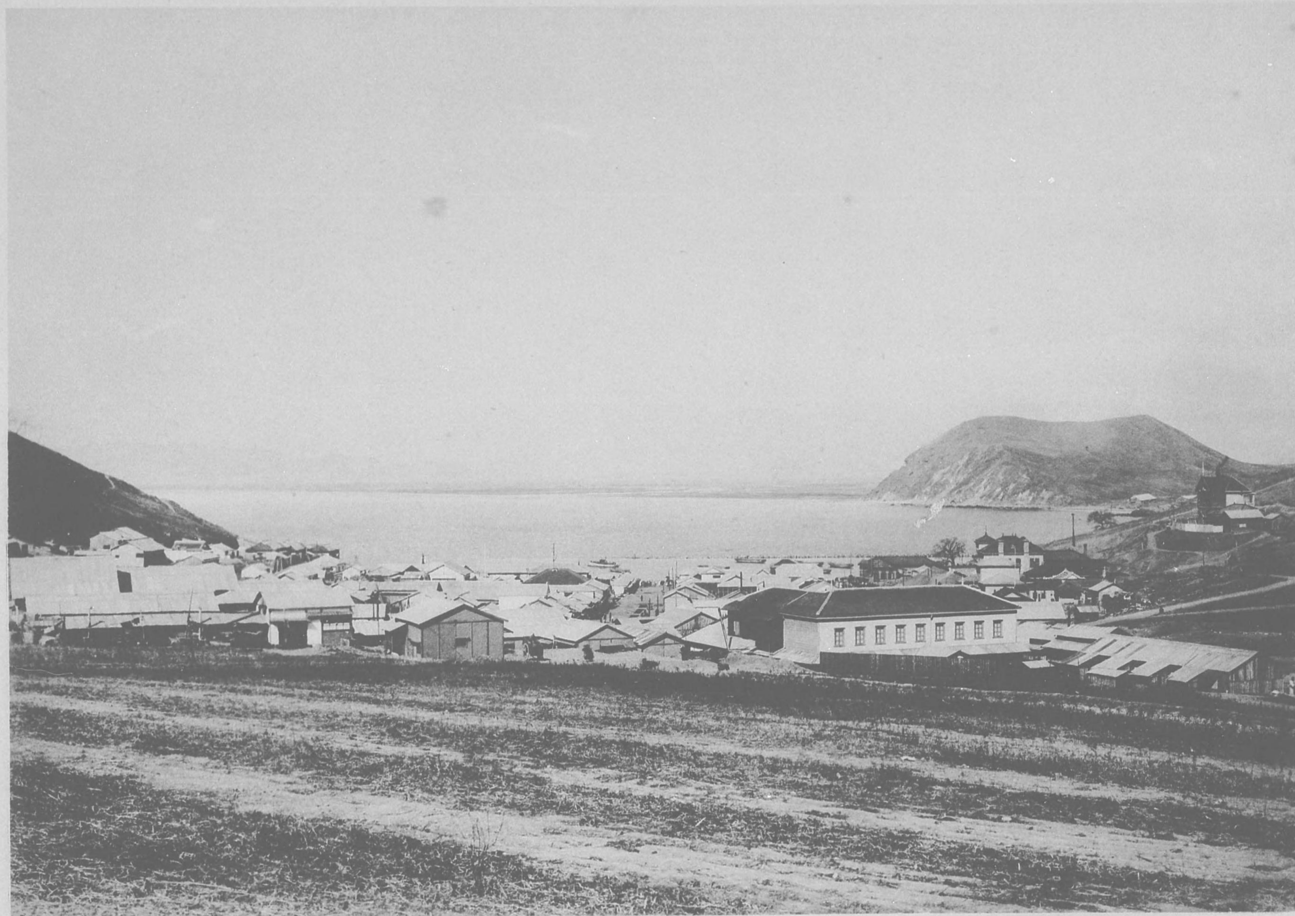
港 津 清 View of the Chong-jin Harbour.
