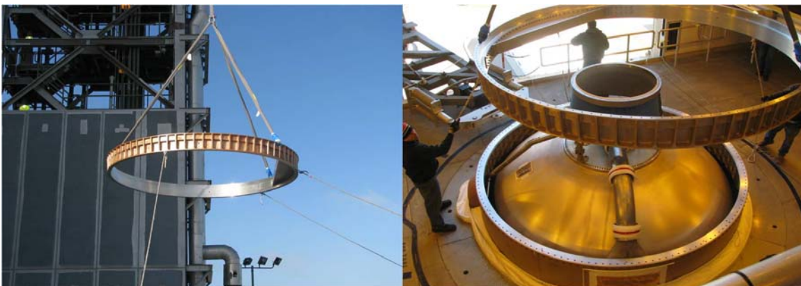
Figure 26. Booster Interstage Adapter Mate
