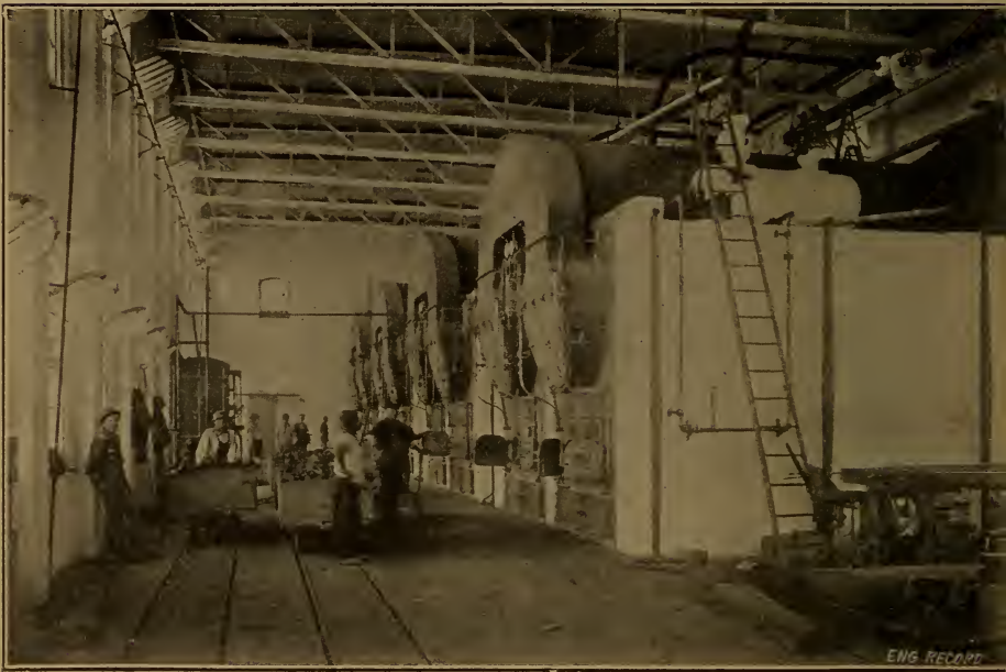
FIGURE 17.—BOILER ROOM PLYMOUTH CORDAGE COMPANY.
