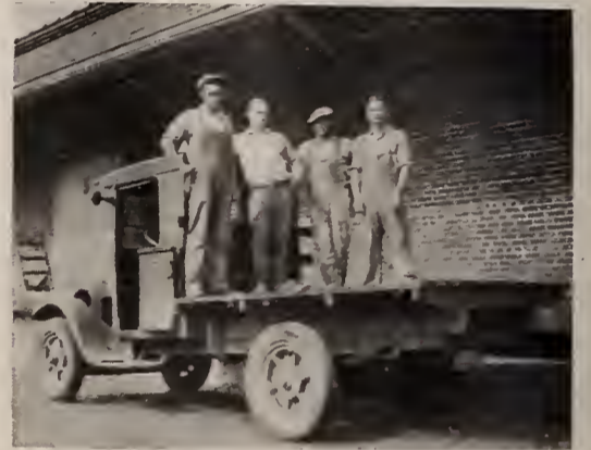
ONE OF THE TRUCKS WITH CREW
