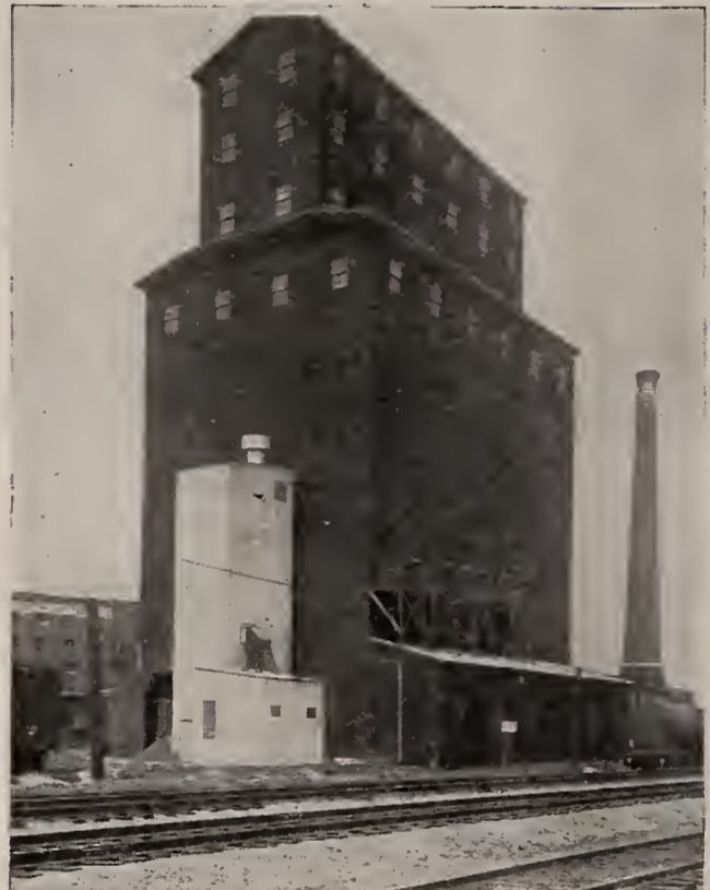
Davenport Elevator Company, Davenport, Iowa.
