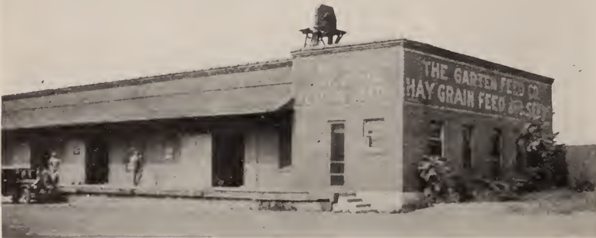
GARTEN FEED COMPANY'S PLANT, INDIANAPOLIS, IND.
