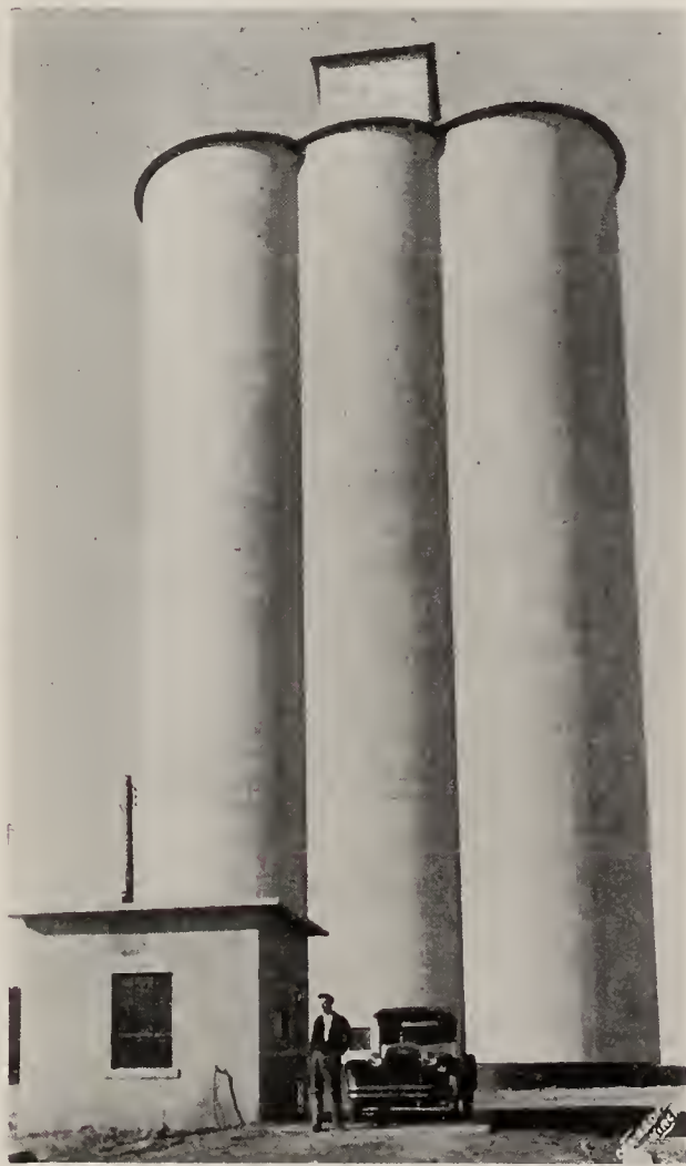
HASKELL COUNTY GRAIN COMPANY'S ELEVATOR AT SUBLETTE, KAN.
