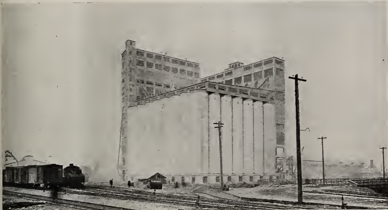
PART OF VANCOUVER'S IMMENSE GRAIN HANDLING FACILITIES
