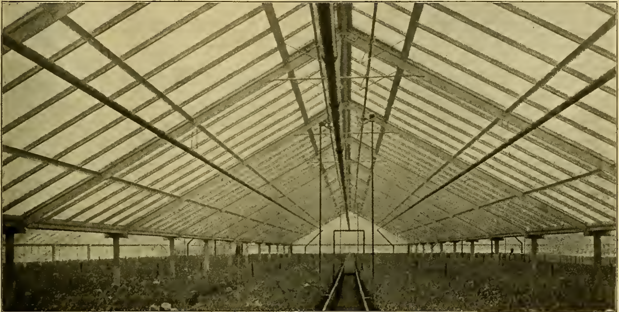
THE ABOVE ILLUSTRATES OUR IRON CONSTRUCTION WITH IRON CUTTER, MADE IN LENGTHS UP TO 25 FEET. FROM A PHOTOGRAPH OF THE CRESSBROOK GREENHOUSES, FALL RIVER, MASS.
